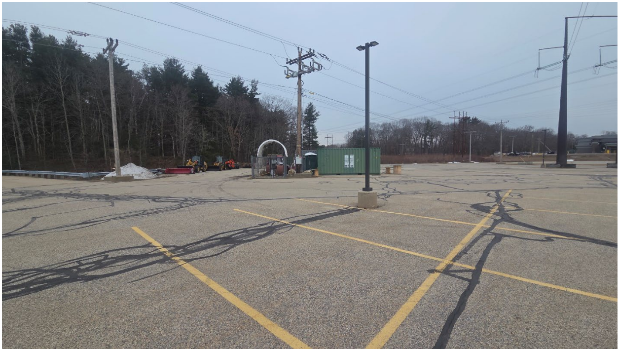
Photo 2 – Liberty Mutual – View looking southwest at the maintenance area (Photo taken 3/20/2026).
