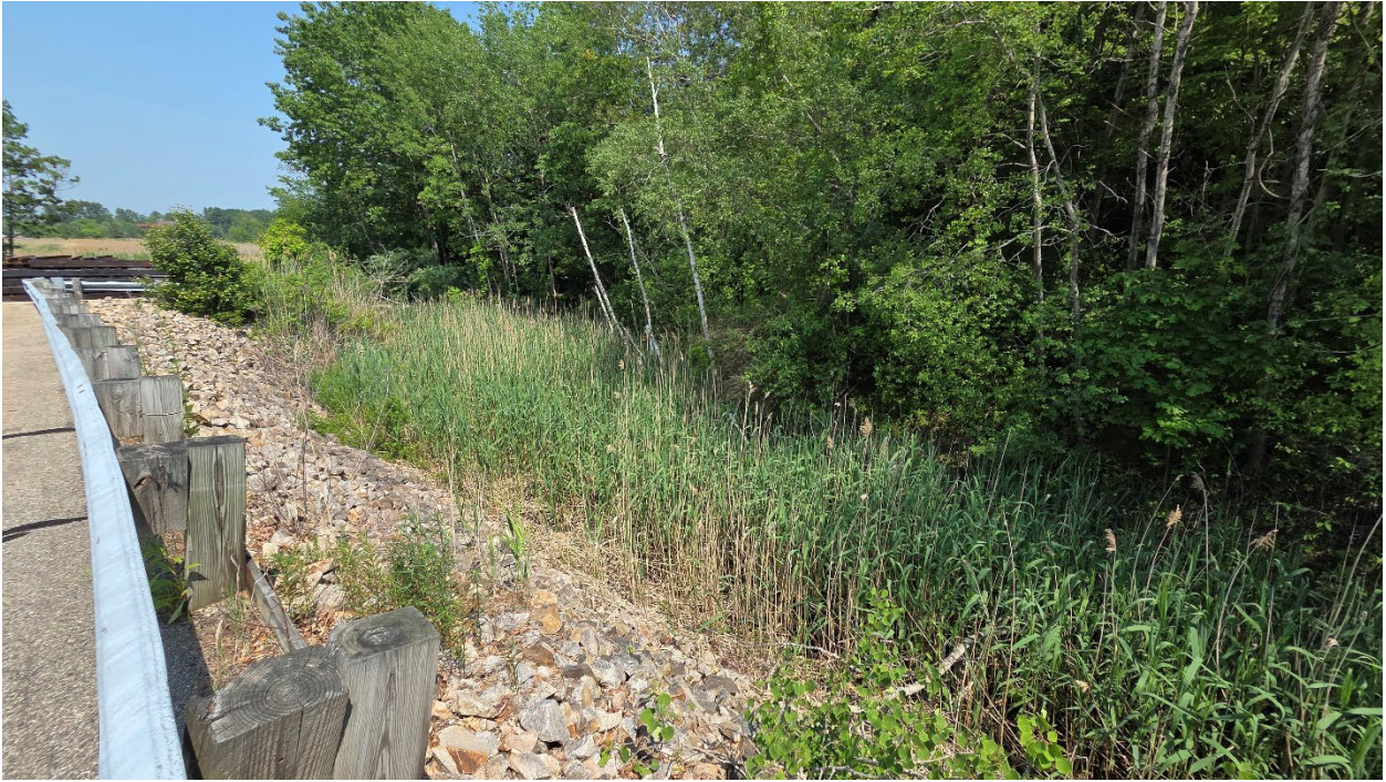
Photo 13 – Liberty Mutual – View looking east along the Stormwater Area (Photo taken 6/5/2025).
