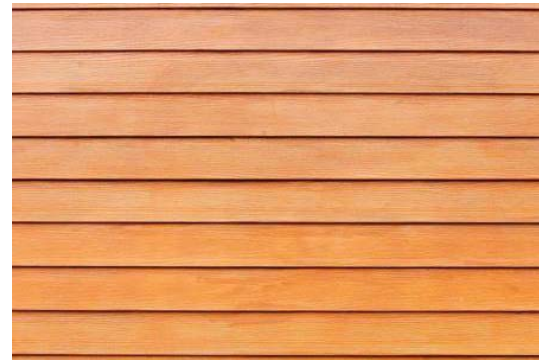
WOOD CLAPBOARD SIDING
