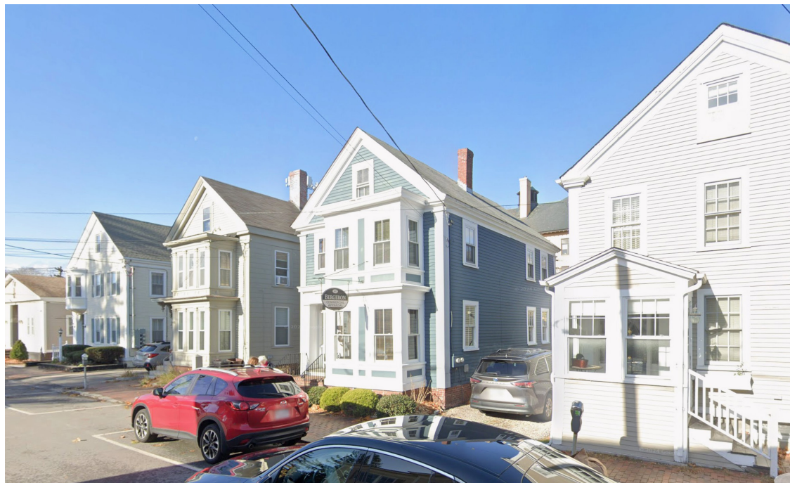
Box Bays and Entry Elements at 481 State St, Portsmouth
