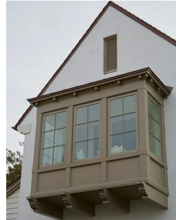
Minimal Panel Box Bay
