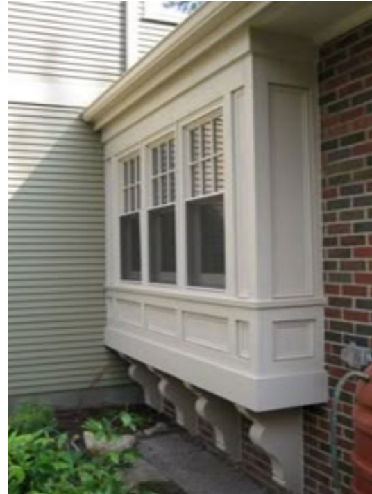
Raised Panel Box Bay
