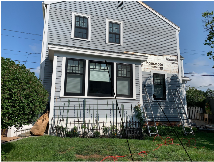
Views of finished Rear Addition
