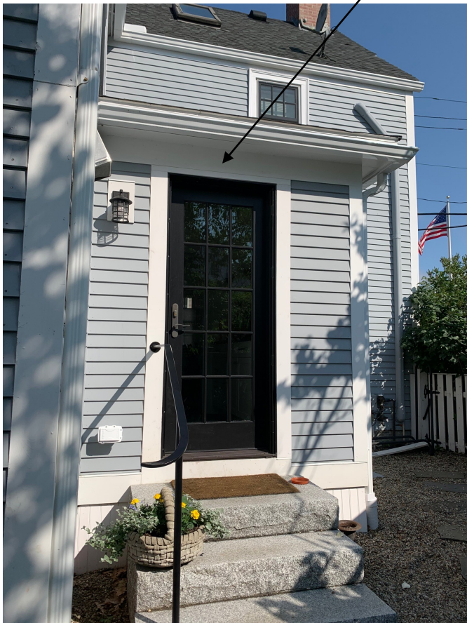
Views of finished Left Side Rear Addition
