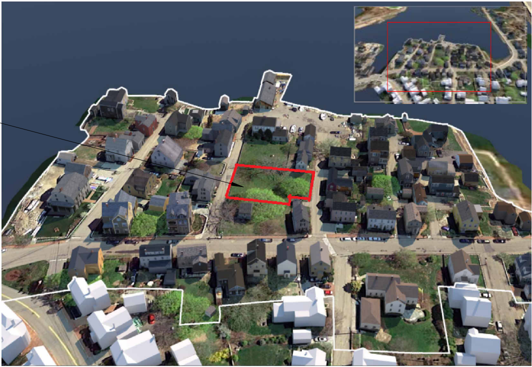
Pray Street Residence 6/13/2025
