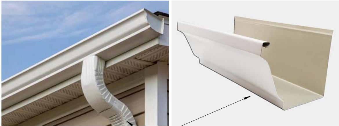
K-STYLE GUTTER AND RECTANGULAR DOWNSPOUT TO MATCH EXISTING
