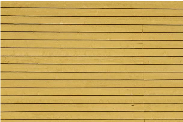
CLAPBOARD SIDING 4" EXPOSURE TO MATCH EXISTING
