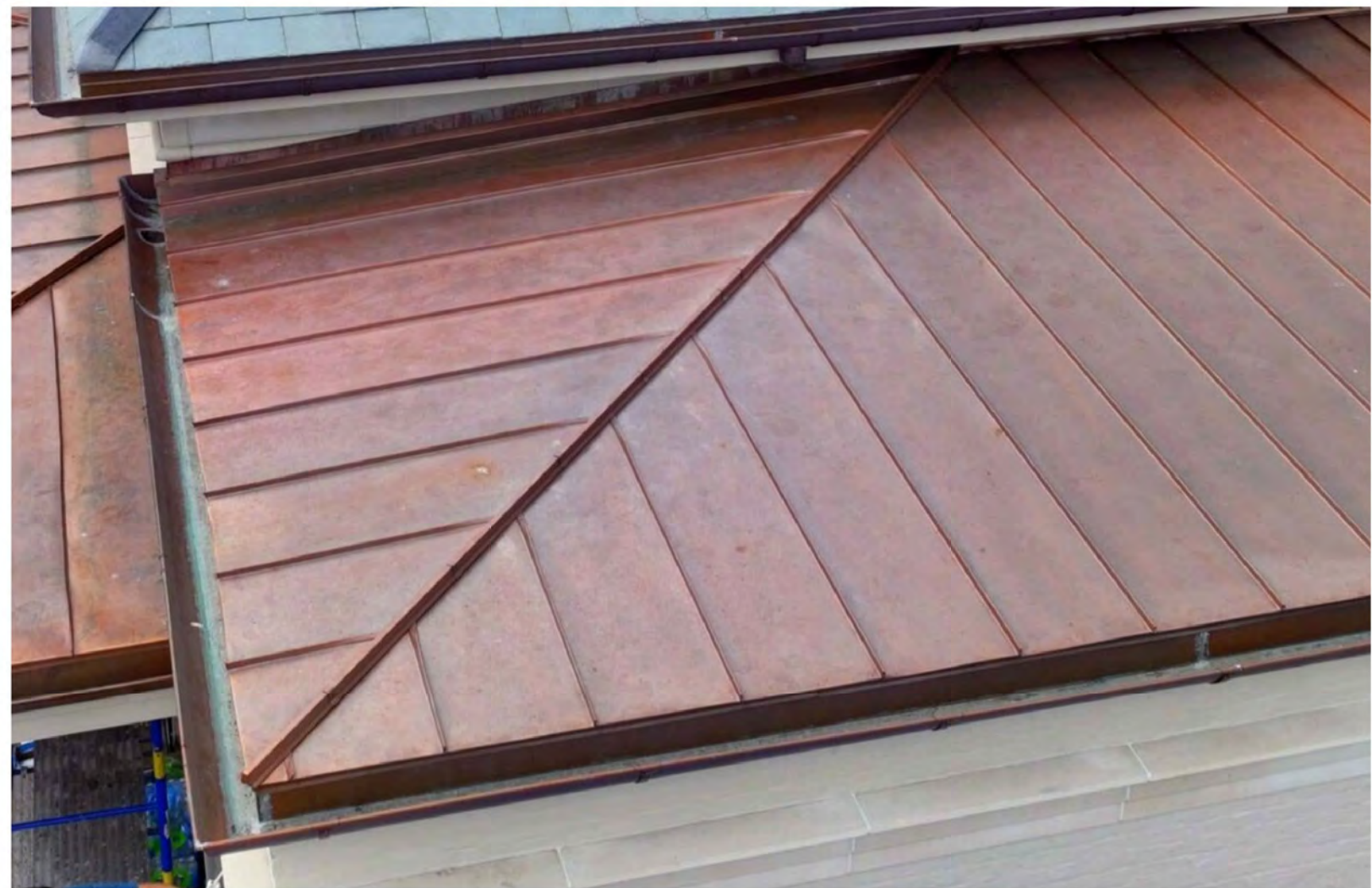
COPPER ROOFING REVERE - CLASSIC COPPER, MILL FINISH, STANDING SEAM
