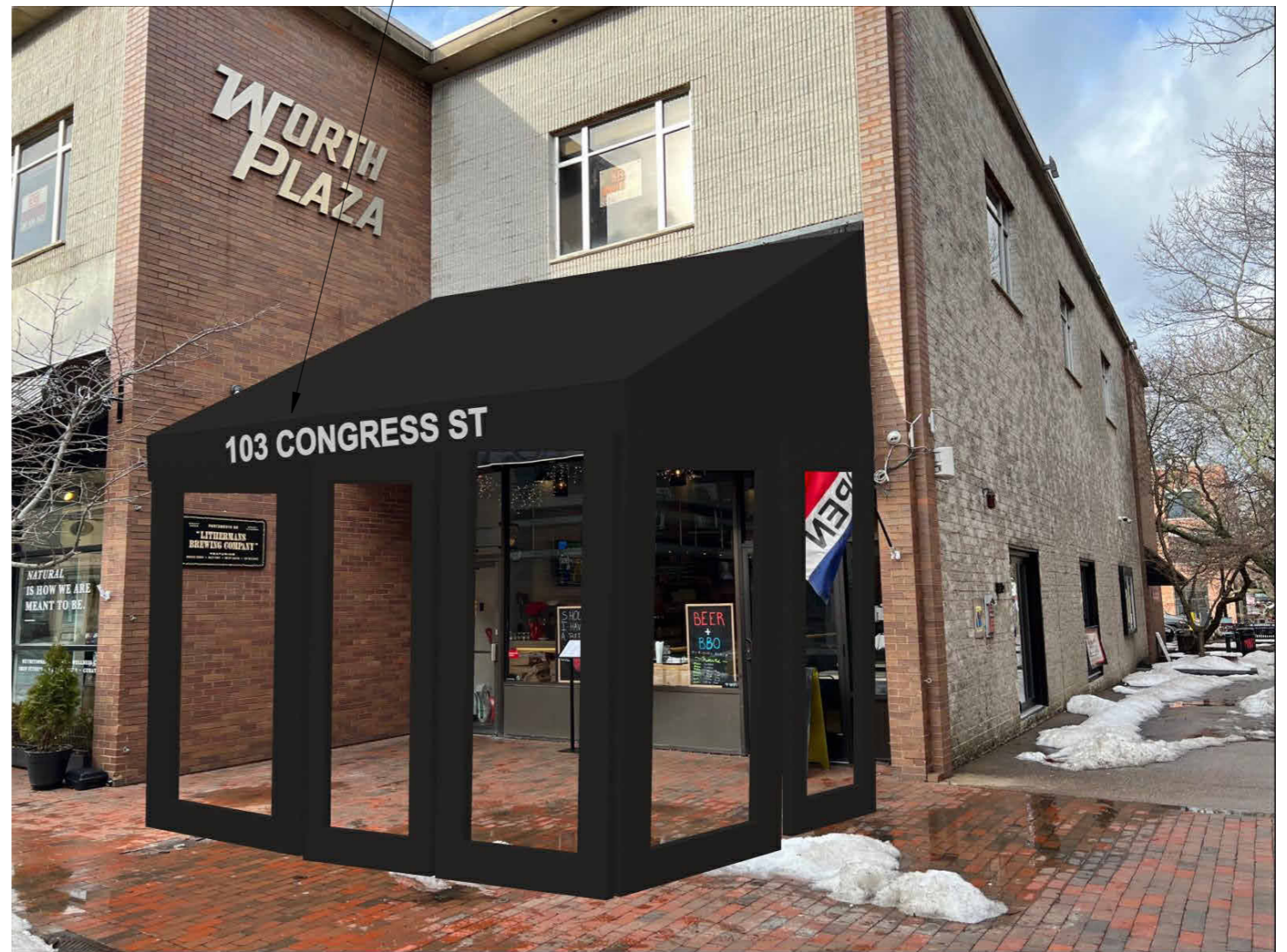
PROPOSED CANOPY - CANVAS CLAD CANOPY ENCLOSURE W/ TRANSLUCENT VINYL DROP-DOWN PANELS "REPLACEMENT IN-KIND" - CONCEPTUAL RENDERING
