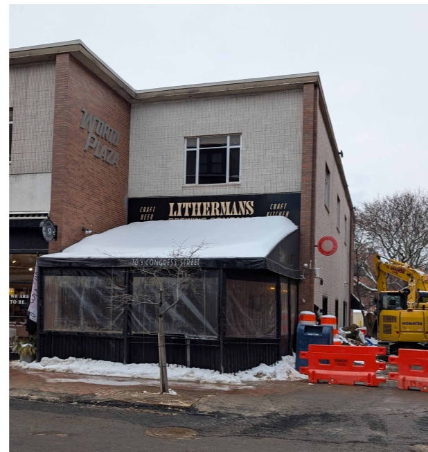
EXISTING EXTERIOR CANOPY PHOTO
