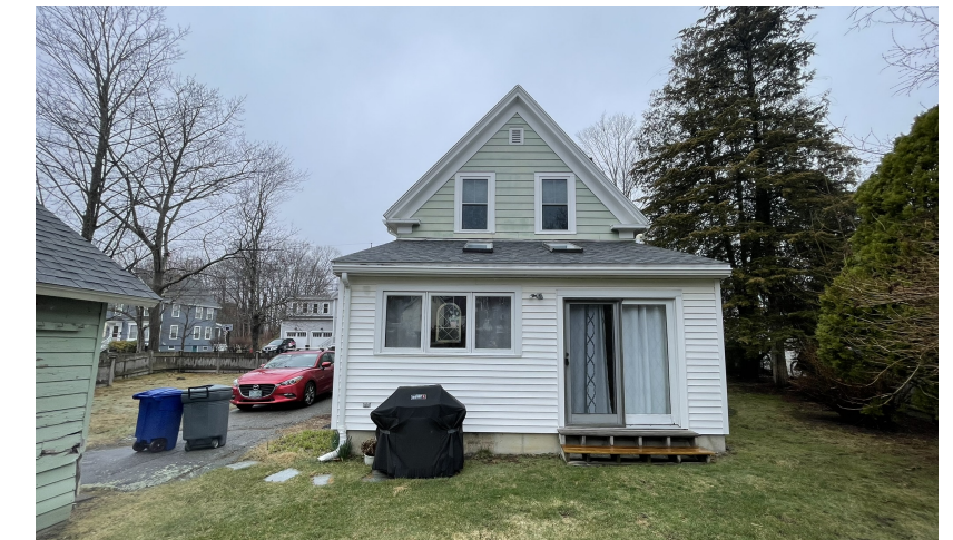
EXISTING REAR OF MAIN HOUSE
