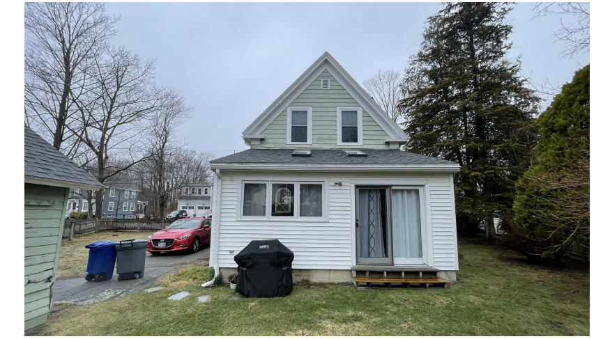
EXISTING REAR OF MAIN HOUSE
