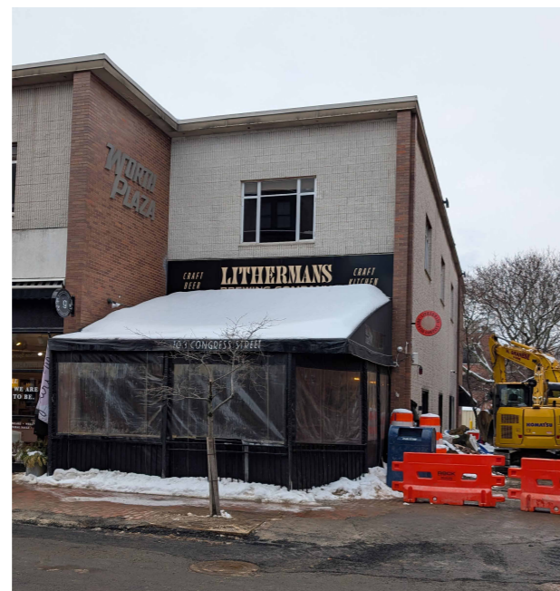
EXISTING EXTERIOR CANOPY PHOTO
