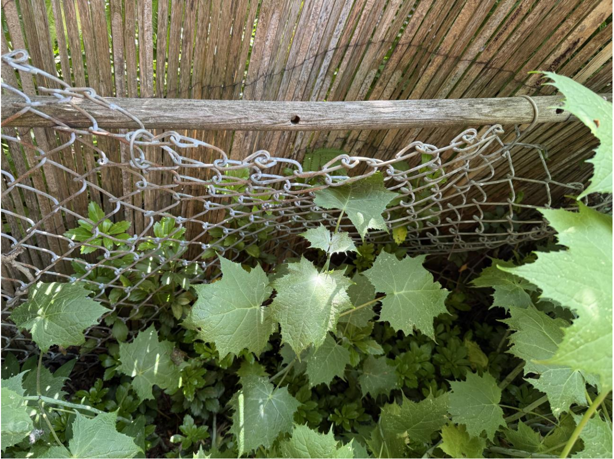
Existing chain-link fencing to be replaced with wood scalloped fencing.
