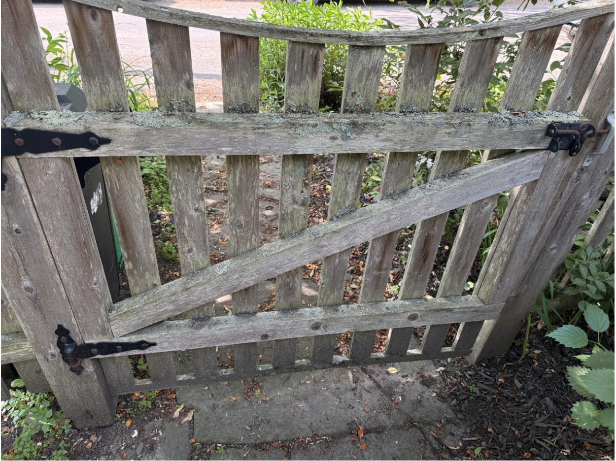
Existing gate to be replaced.
