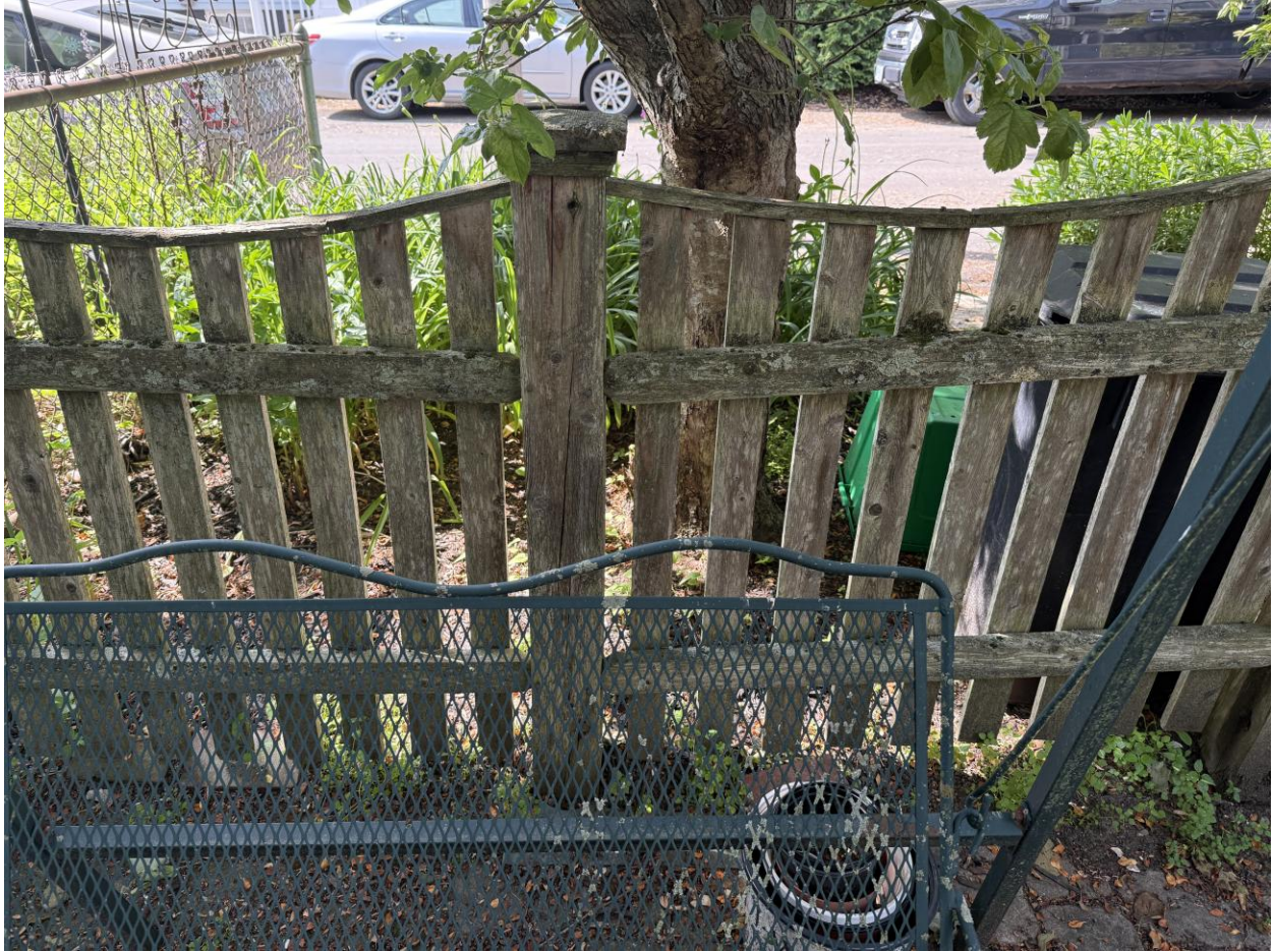
Existing front portion of fencing to be replaced.
