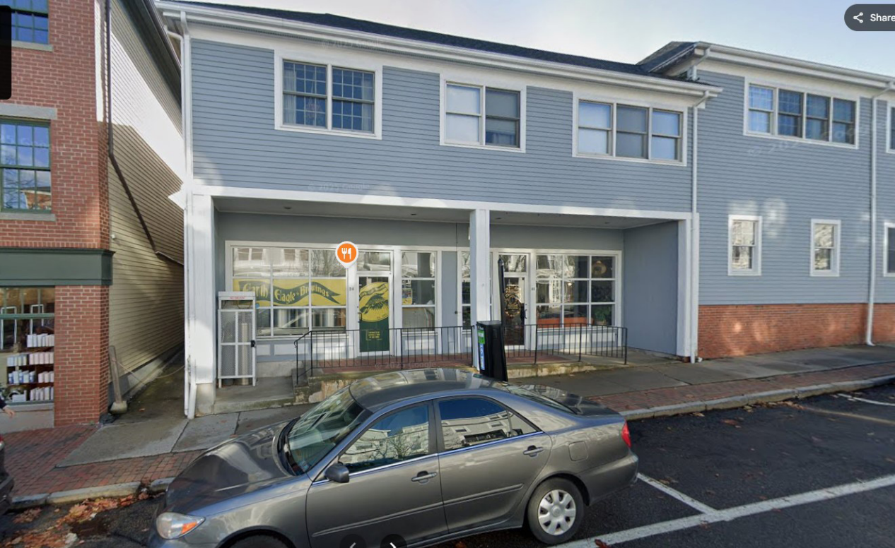
Recessed entry on sloped sidewalk (stair and ramp)
