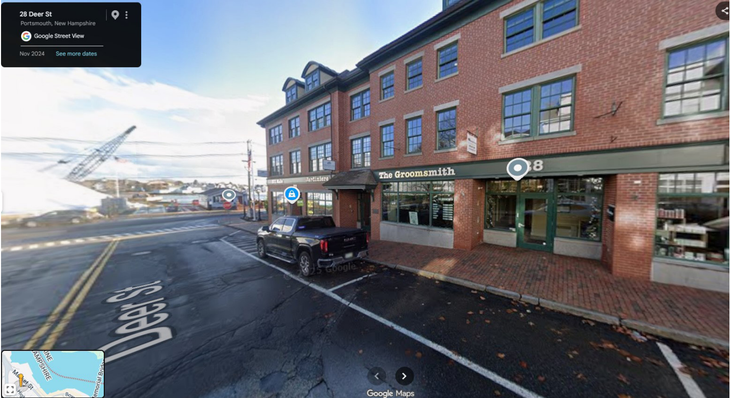
Recessed entry on sloped sidewalk (stair and ramp)
