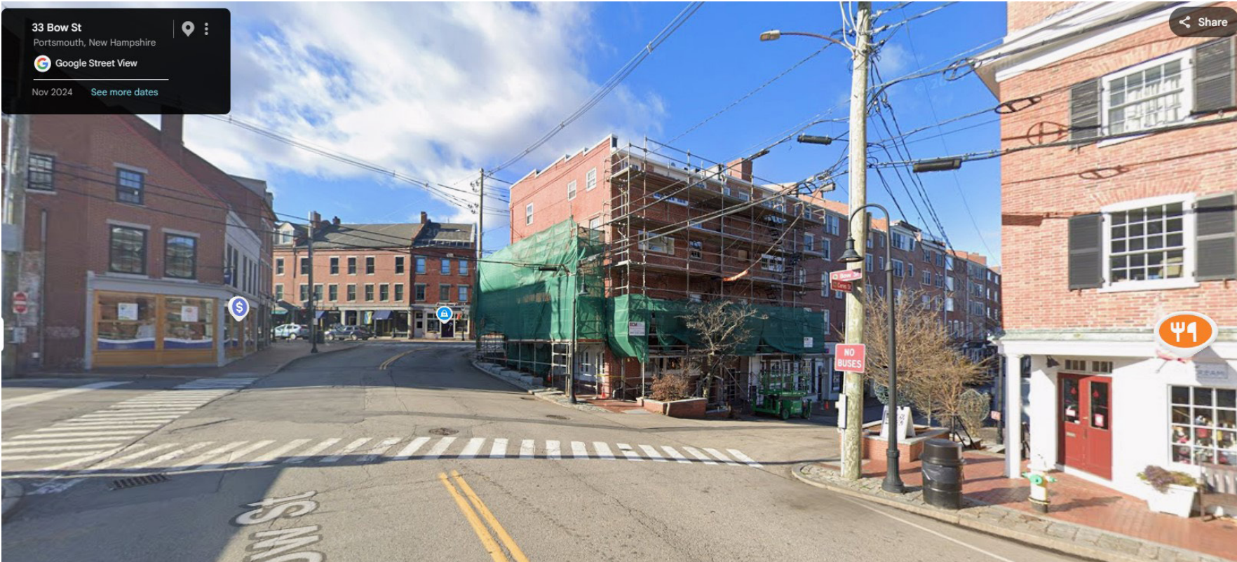
Three different corner treatments on same block
