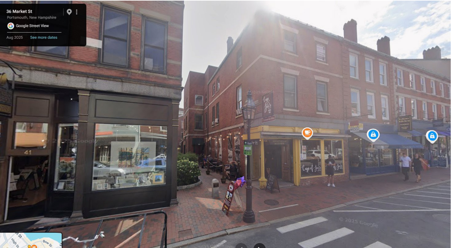
Recessed entry next to public alley
