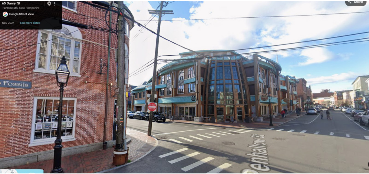
Urban corner anomalies
