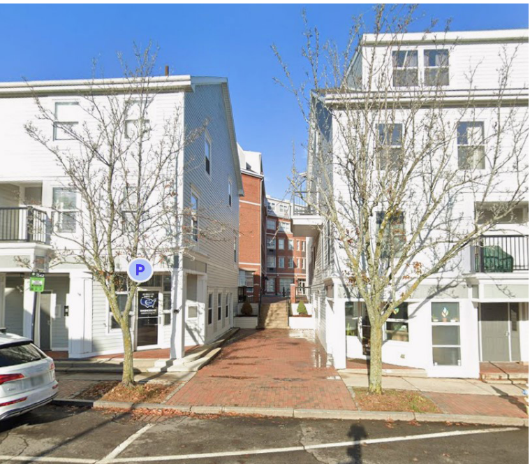
Gaps in street wall
