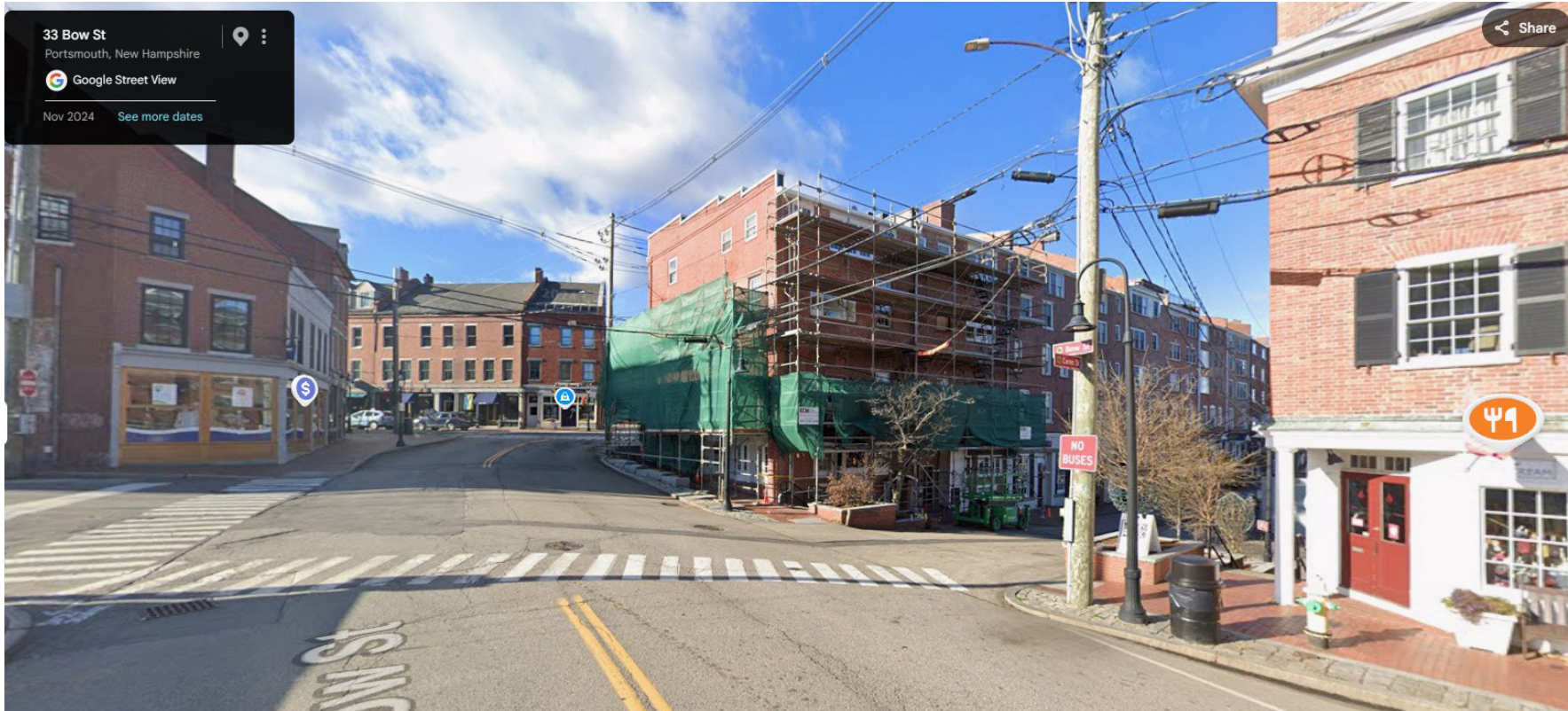
Three different corner treatments on same block
