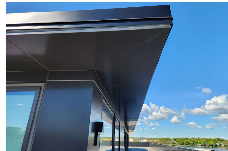
AS-BUILT PENTHOUSE EAVE DETAIL
