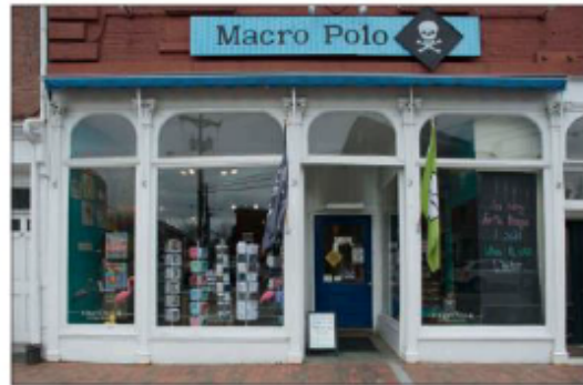
A common feature of many commercial properties in Portsmouth is a storefront. This example includes arched transoms, a recessed entrance alcove, and decorative supports flanking display windows.
