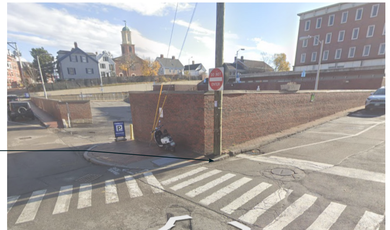
Inaccessible street level
