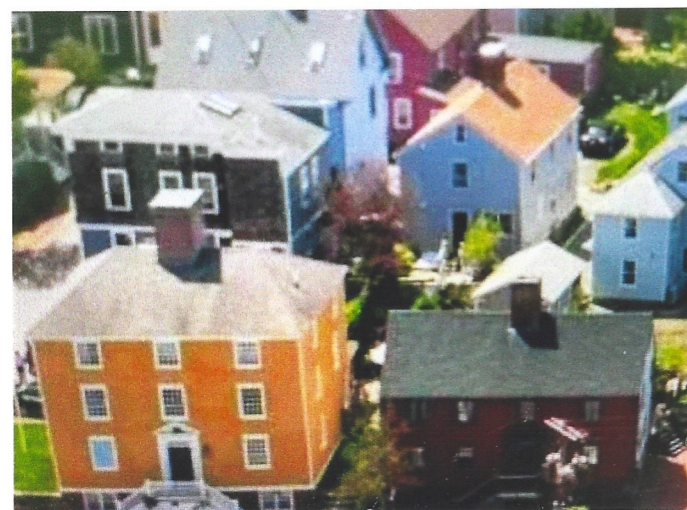
VIEW OF ROOF TOPS
