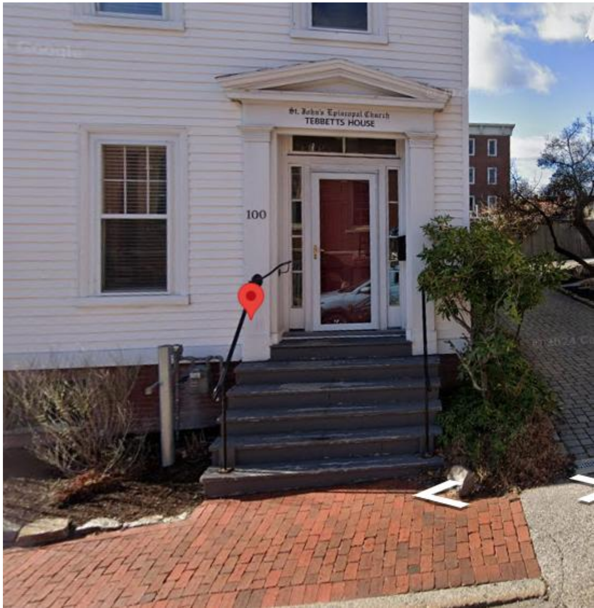
Existing wooden stairs and railings.
