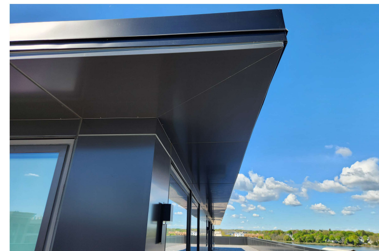
AS-BUILT PENTHOUSE EAVE DETAIL
