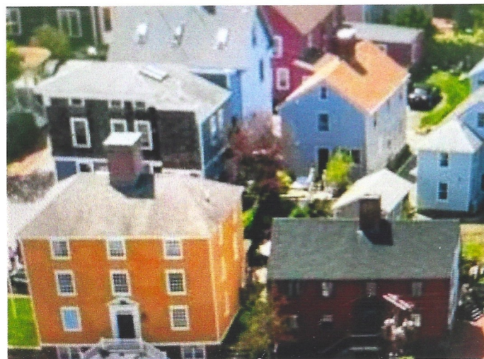
VIEW OF ROOF TOPS
