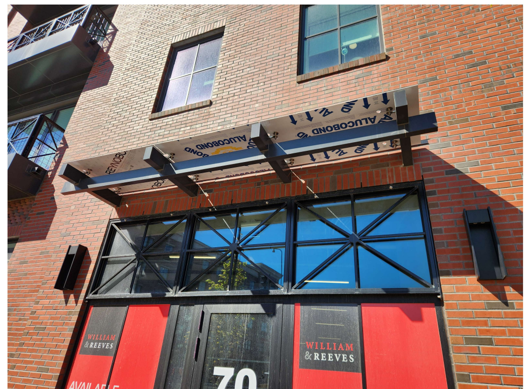
AS-BUILT CANOPIE PHOTO
