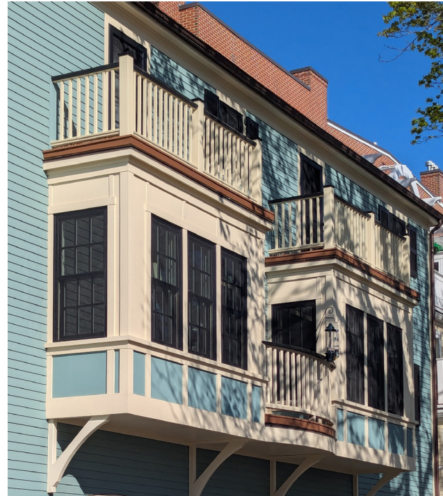
Balcony Box Bay near 461 Court St
