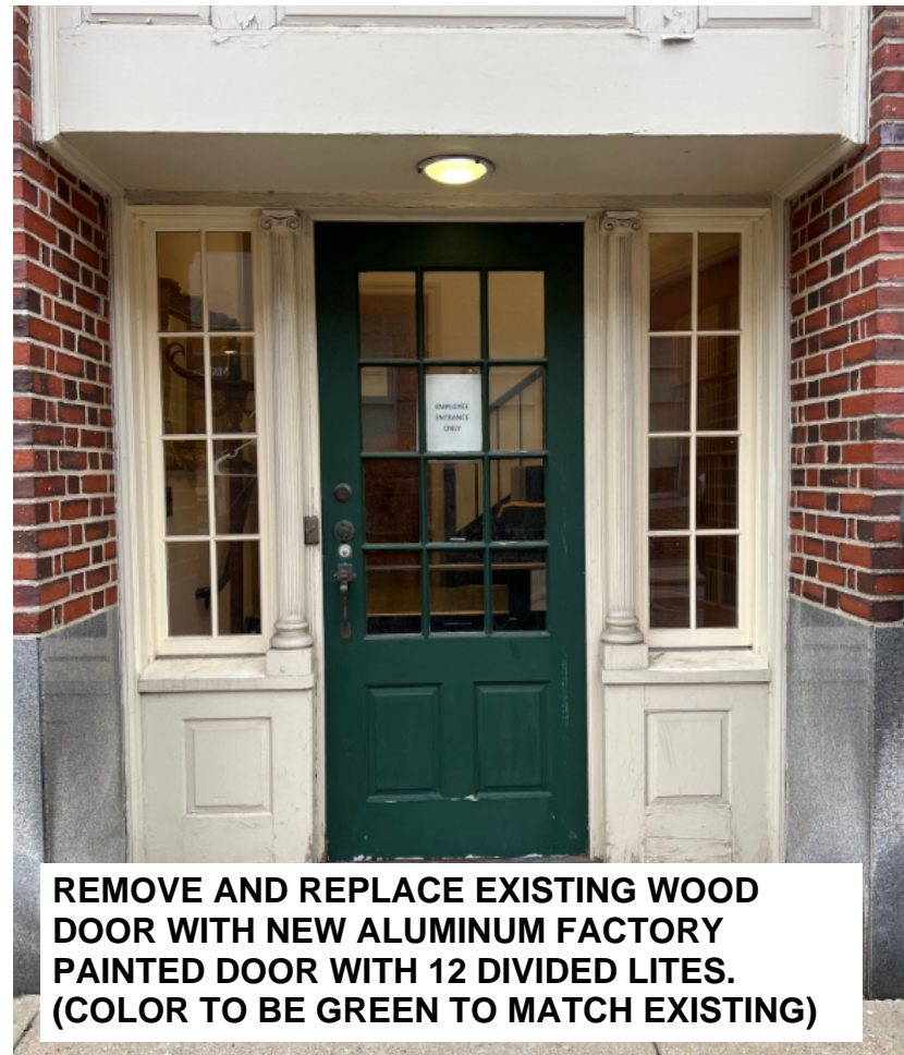
EXISTING DOOR AT OPENING #2
