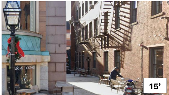
36 – Brick Market Alley (North)
