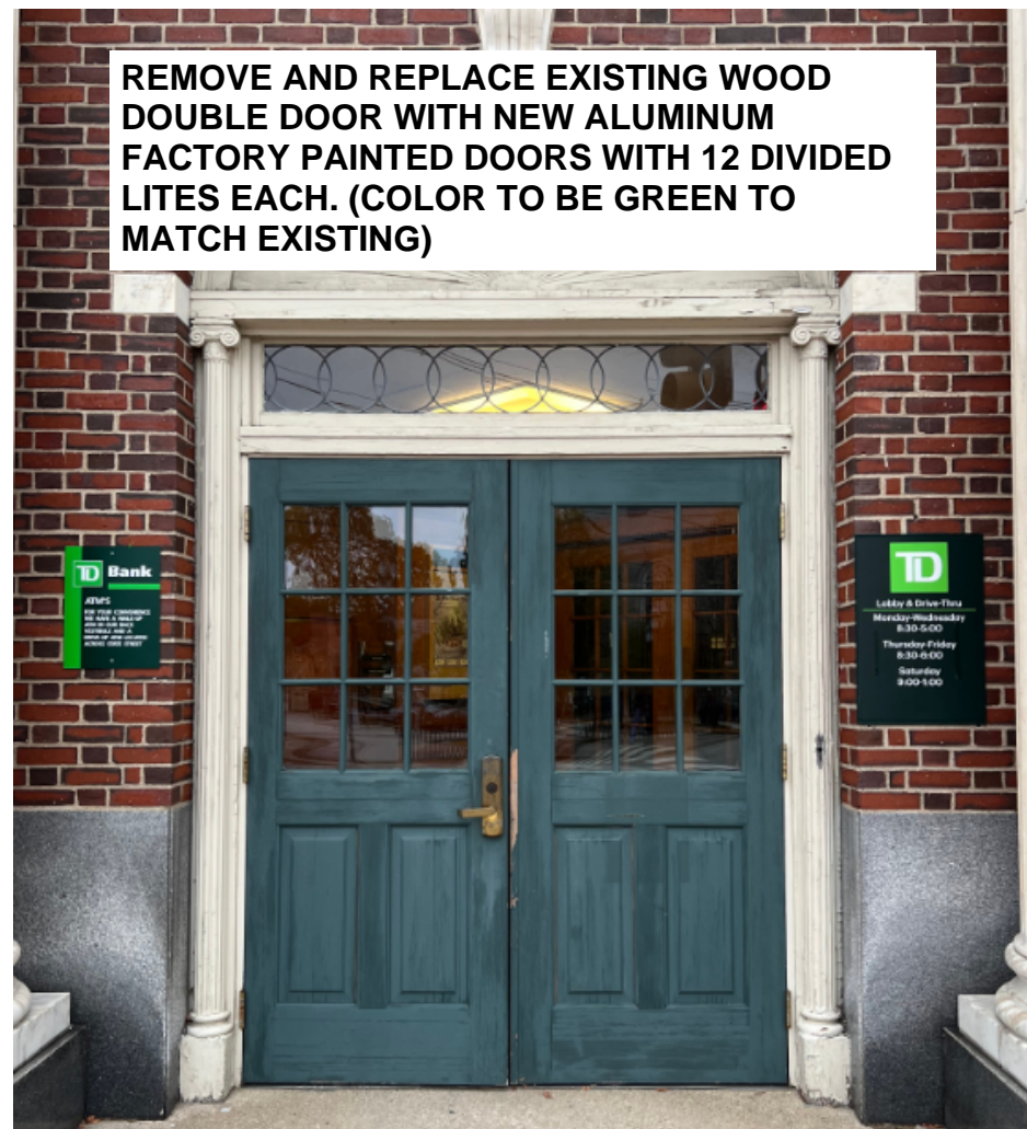
EXISTING DOORS AT OPENING #3
