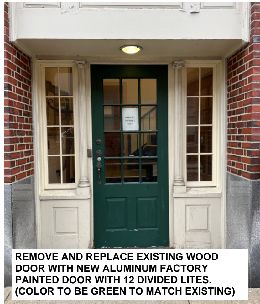
EXISTING DOOR AT OPENING #2
