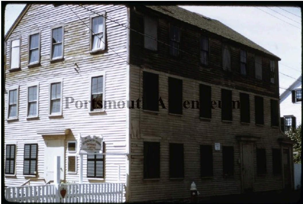
These images from the 1970s (top) and 1980s (bottom) indicate a simple spaced picket fence painted white with a top rail cap and a heavier bottom rail that was installed by SBM.
