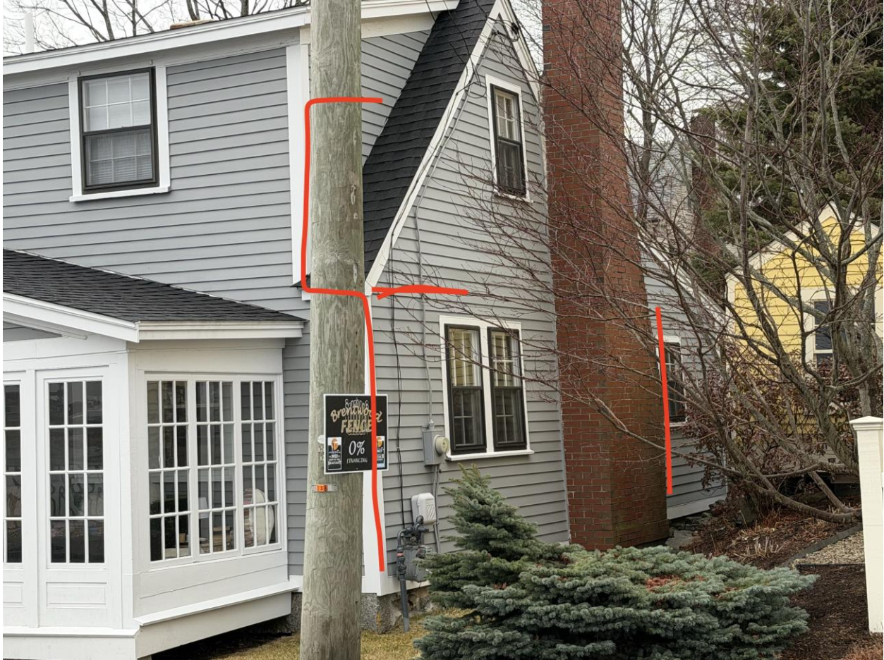
Proposed location(s) of the conduit lines. The conduit lines will be covered.
