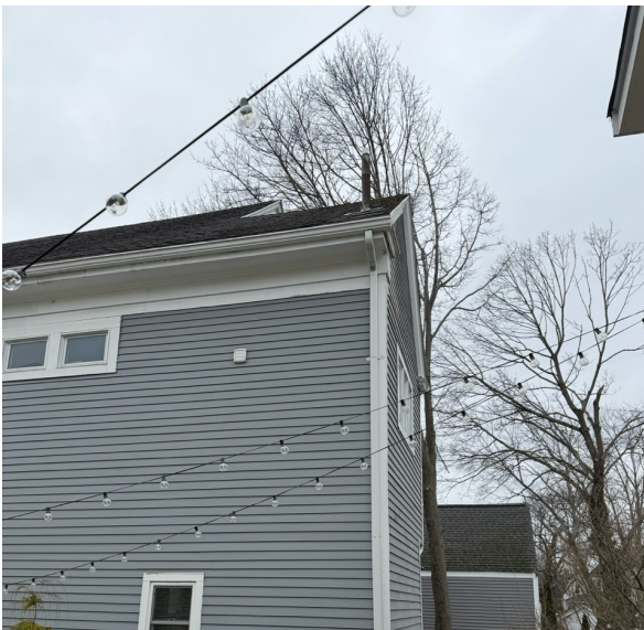
Photo 11 — Adjacent Building (Grey) — White Gutter and downspout for reference
