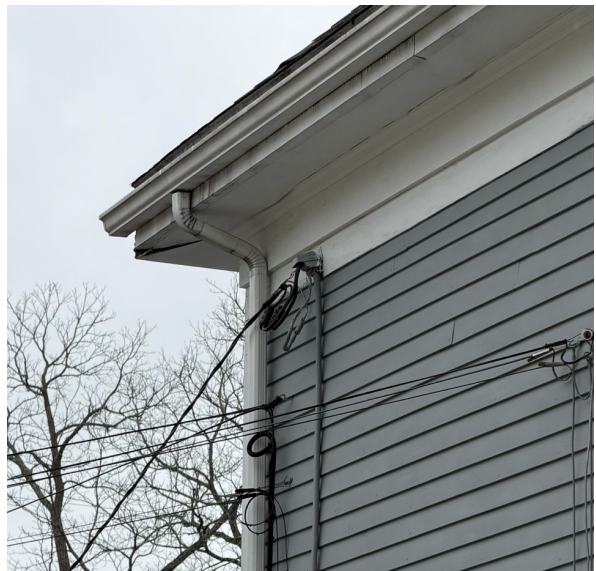
Photo 12 — Adjacent Building (Grey) — White Gutter and downspout for reference
