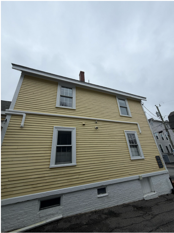
Photo 8 — Main House Rear Elevation & Chimney
