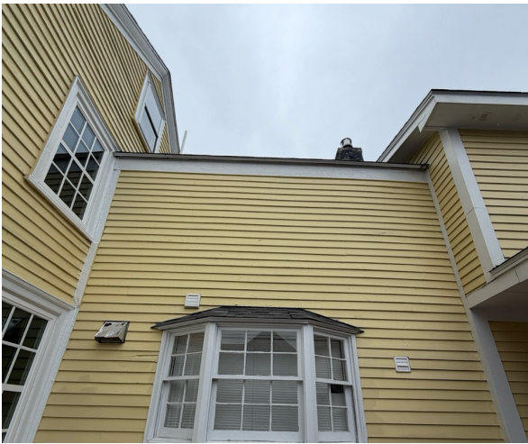
Photo 3 — Rear Elevation: Bay Window & Chimney Detail
