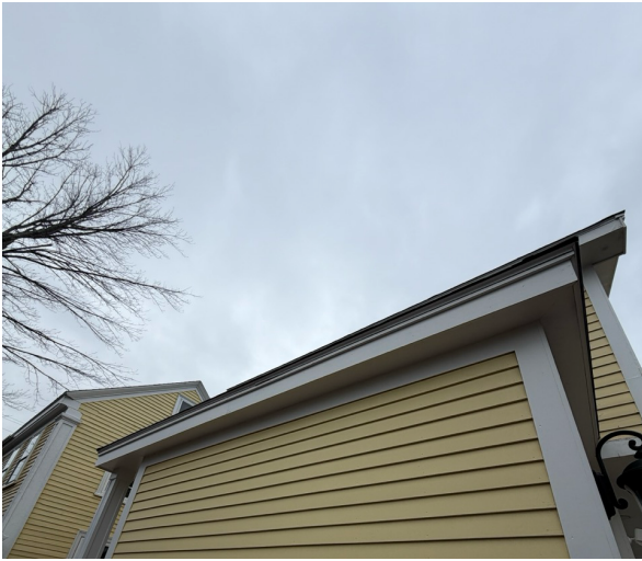
Photo 5 — Roofline & Fascia, Carriage House End Gable
