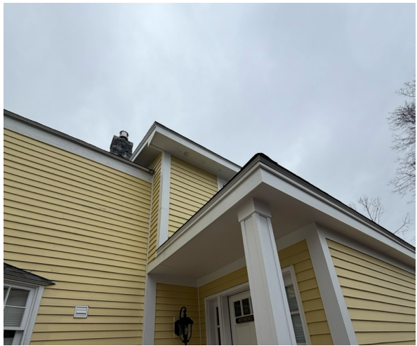
Photo 4 — Athens Suite Entrance Canopy
