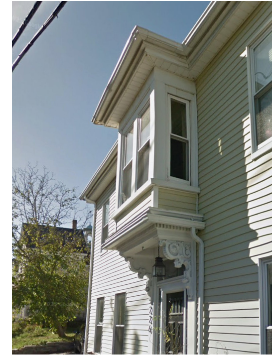
Bay Side Window at 226 NH1B
