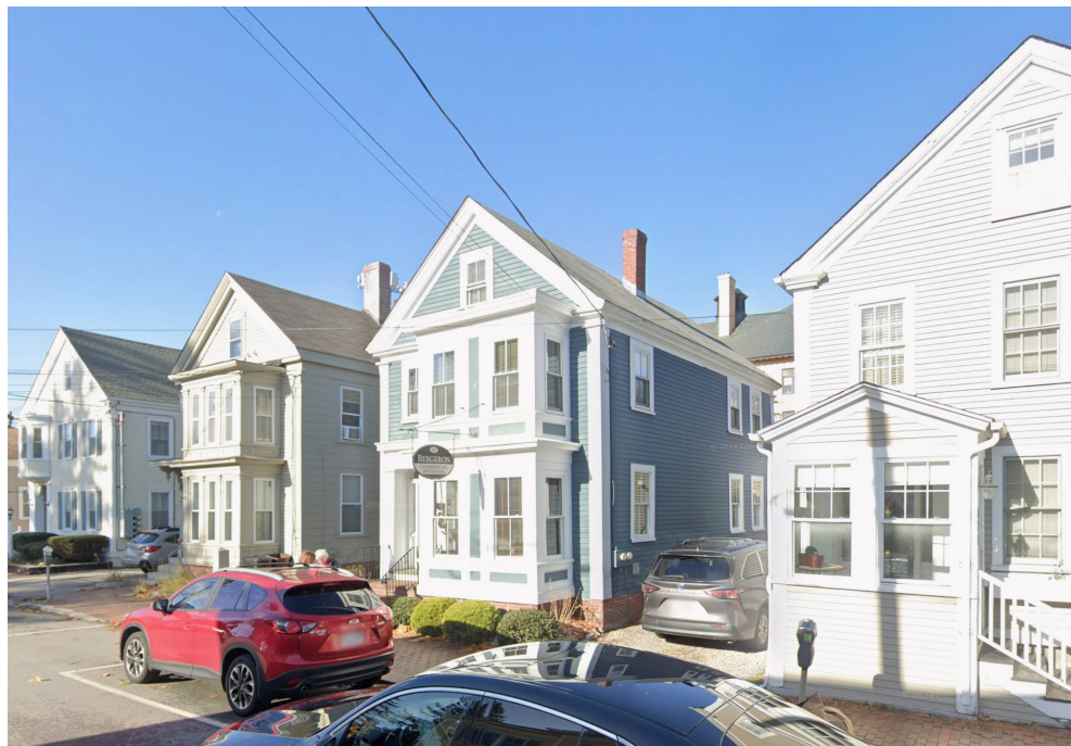
Box Bays and Entry Elements at 481 State St, Portsmouth
