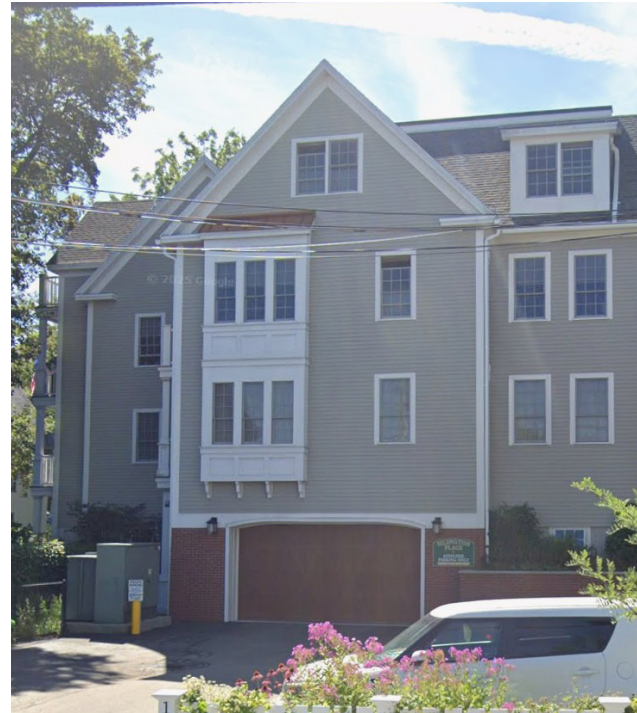
2-Story Box Bay at 198 Islington St
