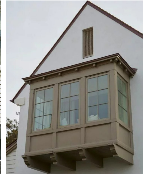
Minimal Panel Box Bay
