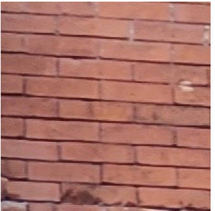
EXISTING BRICK - 15 CONGRESS STREET
