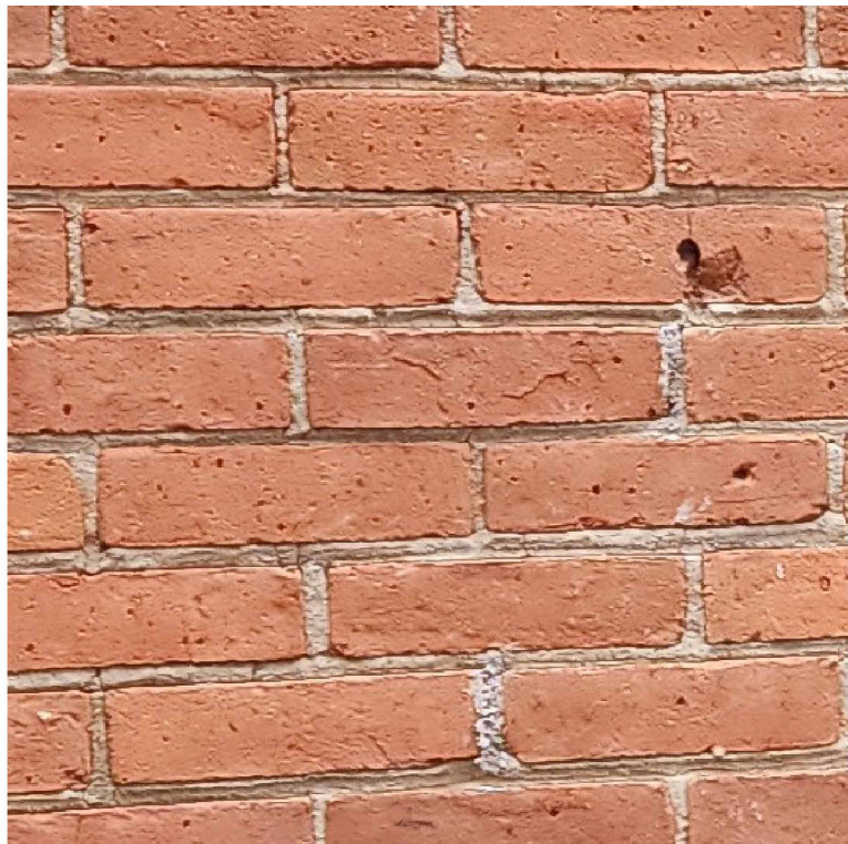
EXISTING BRICK - HAVEN COURT EAST
