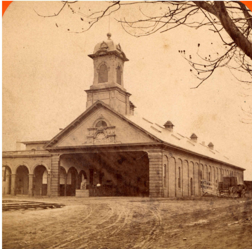
BOSTON & MAINE RAILROAD DEPOT 1864
