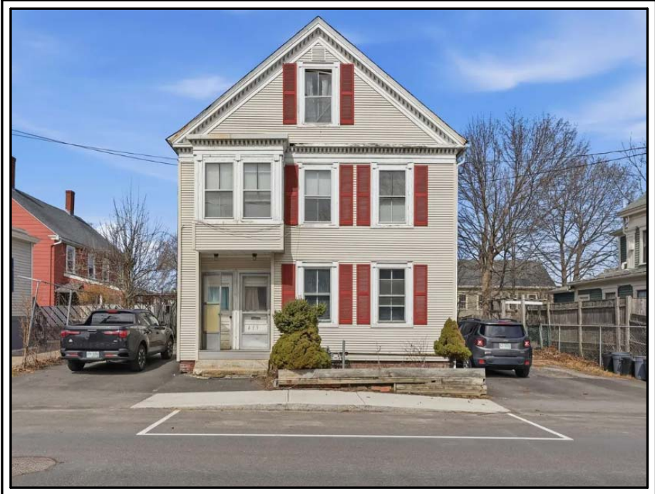
SOUTH VIEW FROM ISLINGTON STREET
