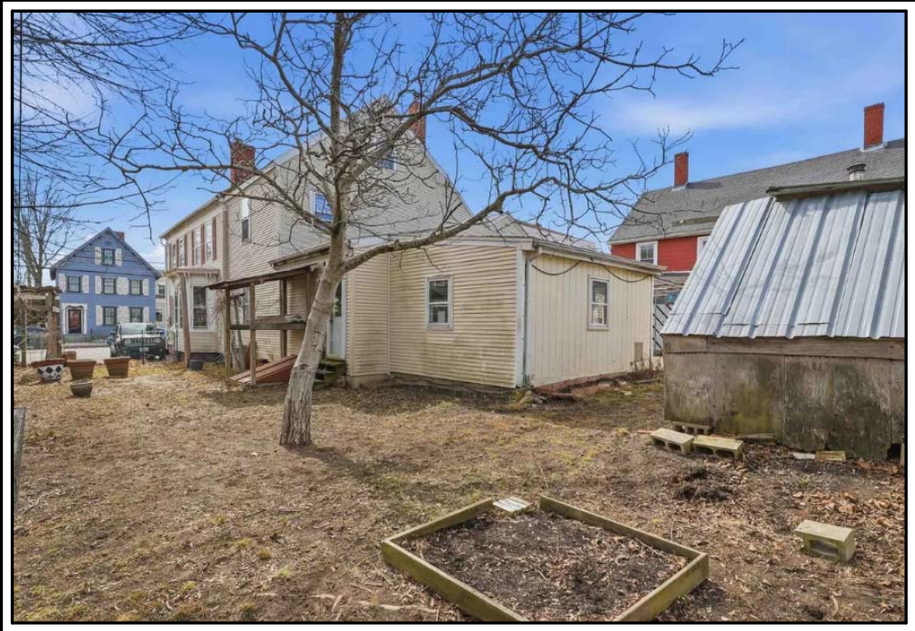
VIEW FROM REAR YARD
