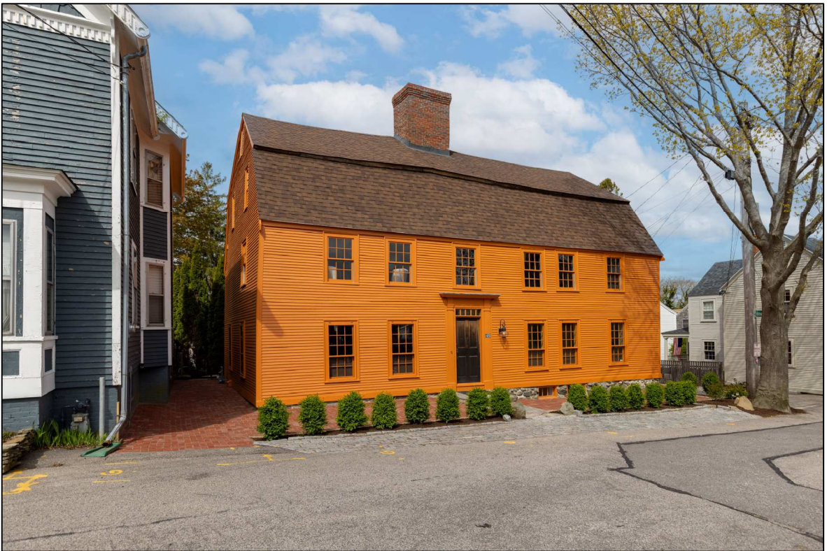
Existing View from Manning Street
