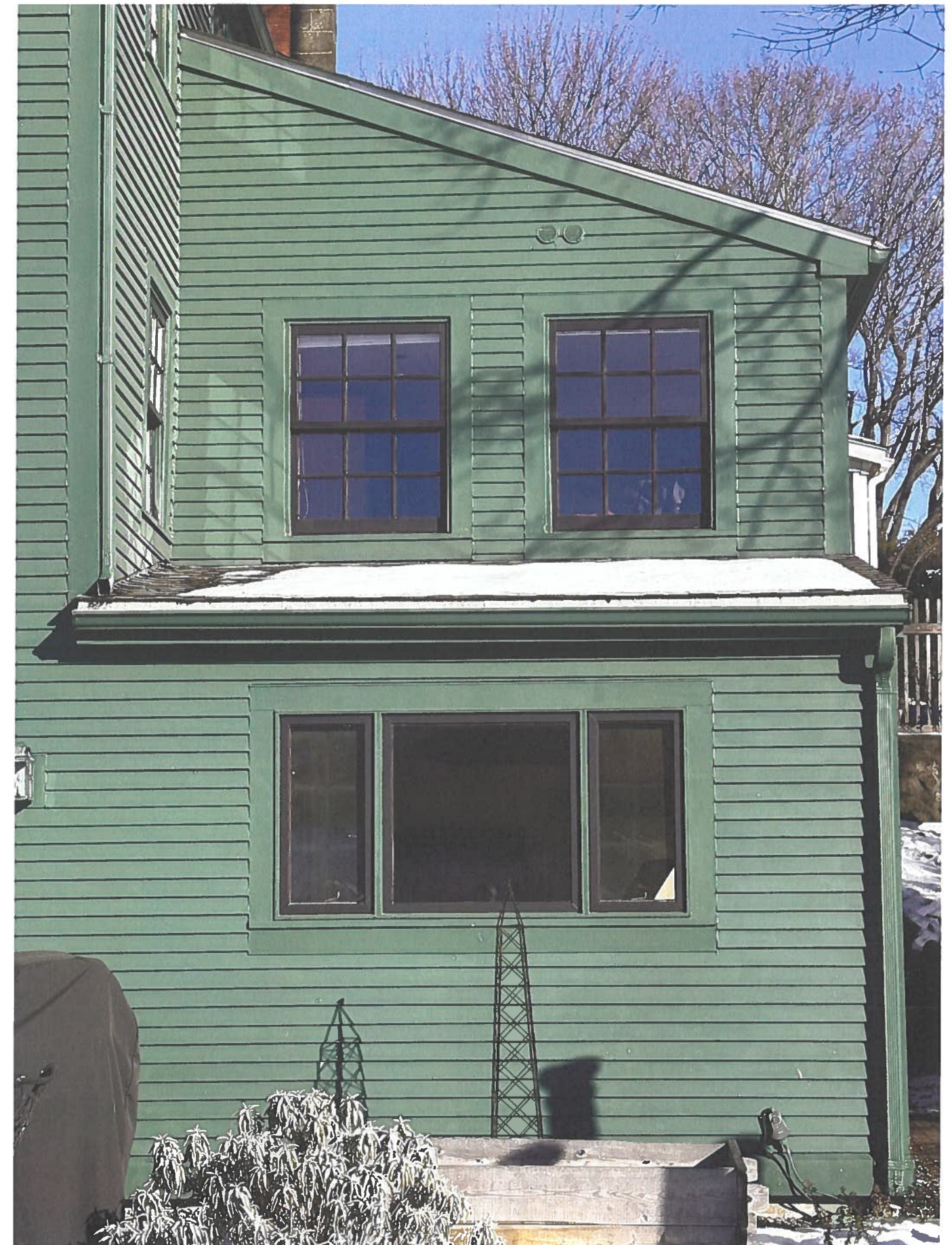
South Elevation: close-up of existing one-story addition
