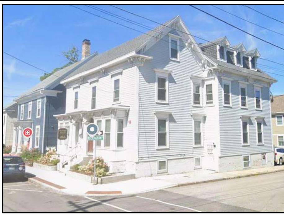
303 ISLINGTON FROM ISLINGTON AND ROCKINGHAM STREET
