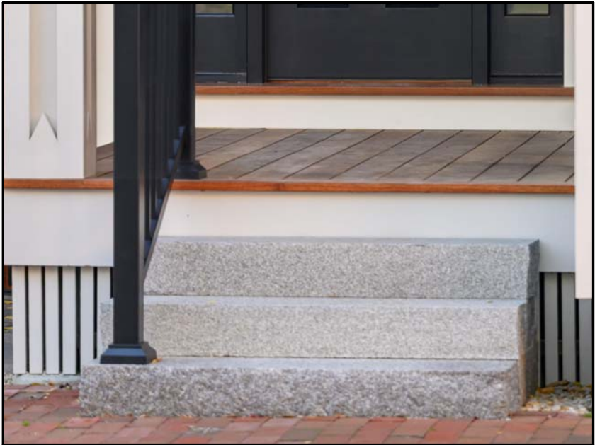
GRANITE FRONT STEPS
