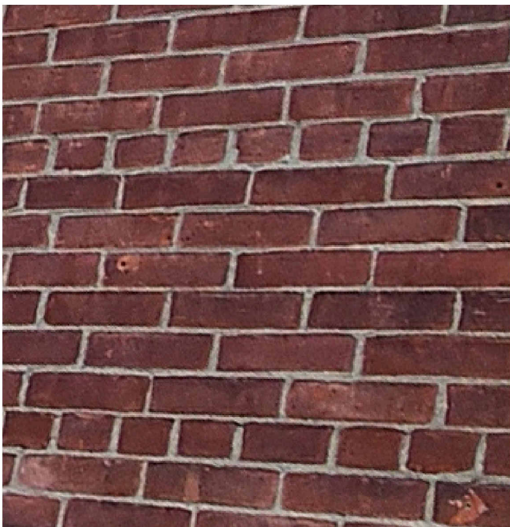
EXISTING BRICK - HAVEN COURT WEST
