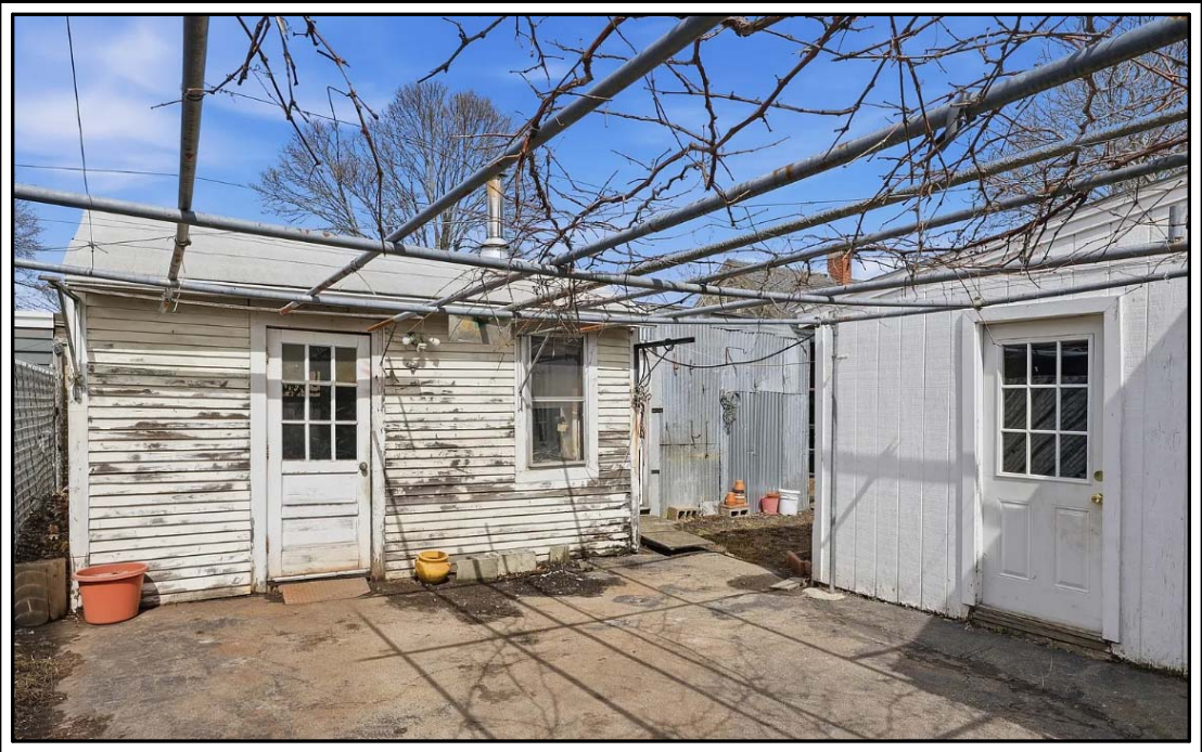
VIEW OF SHED AND REAR OF HOUSE
