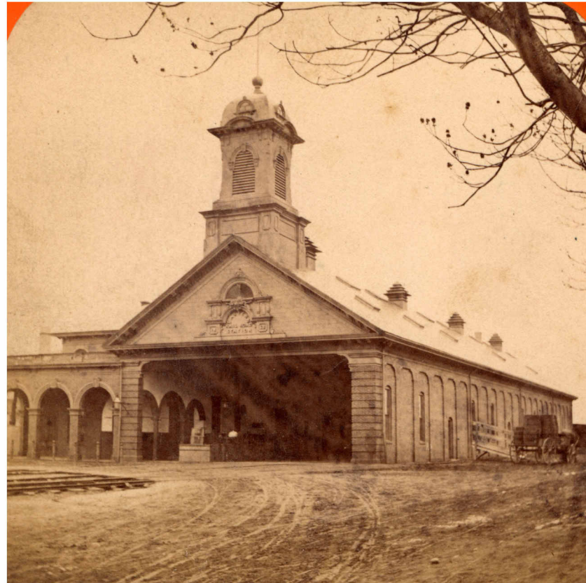
BOSTON & MAINE RAILROAD DEPOT 1864
