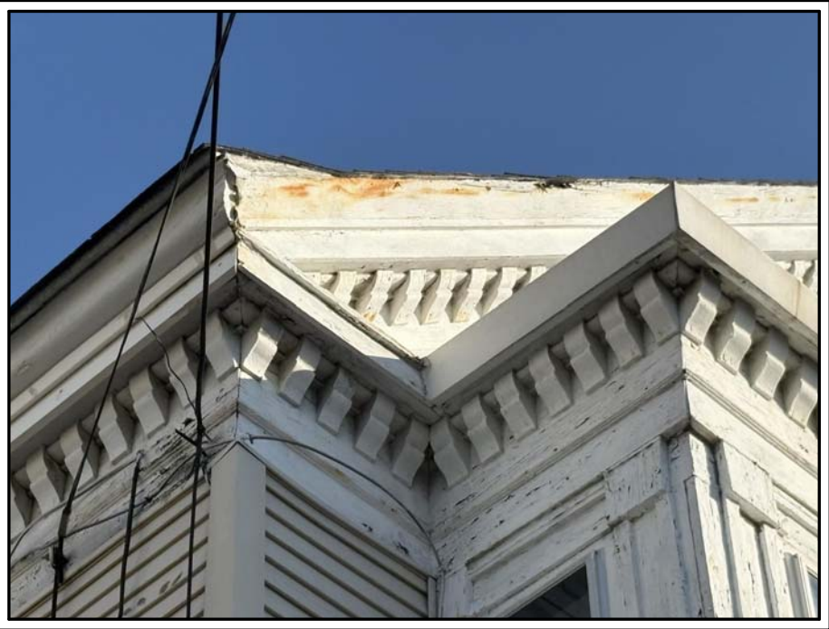
VIEW OF MOLDING, FASCIA, AND TRIM
