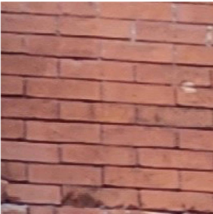
EXISTING BRICK - 15 CONGRESS STREET
