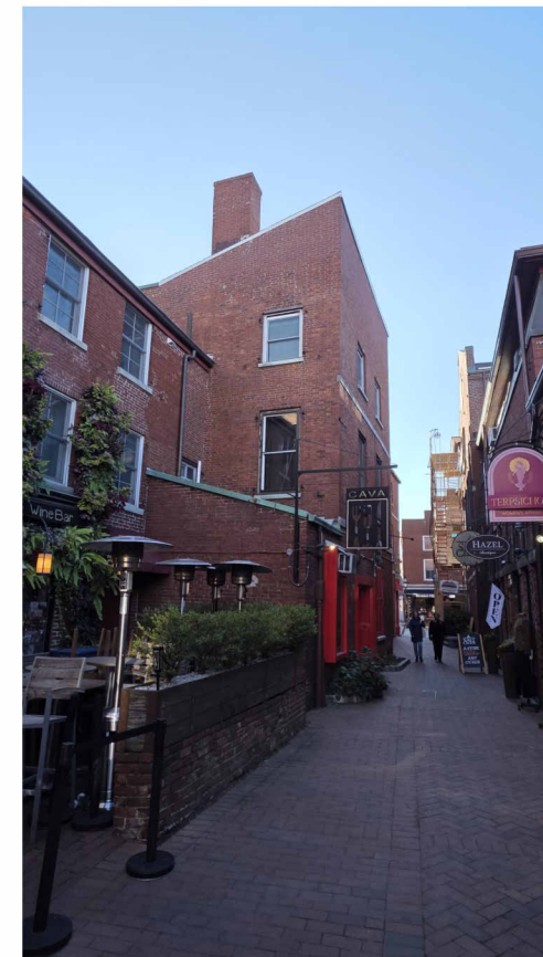
HISTORIC REFERENCE: TYPICAL HISTORIC CORE REAR SKYLINE (COMMERCIAL ALLEY)
