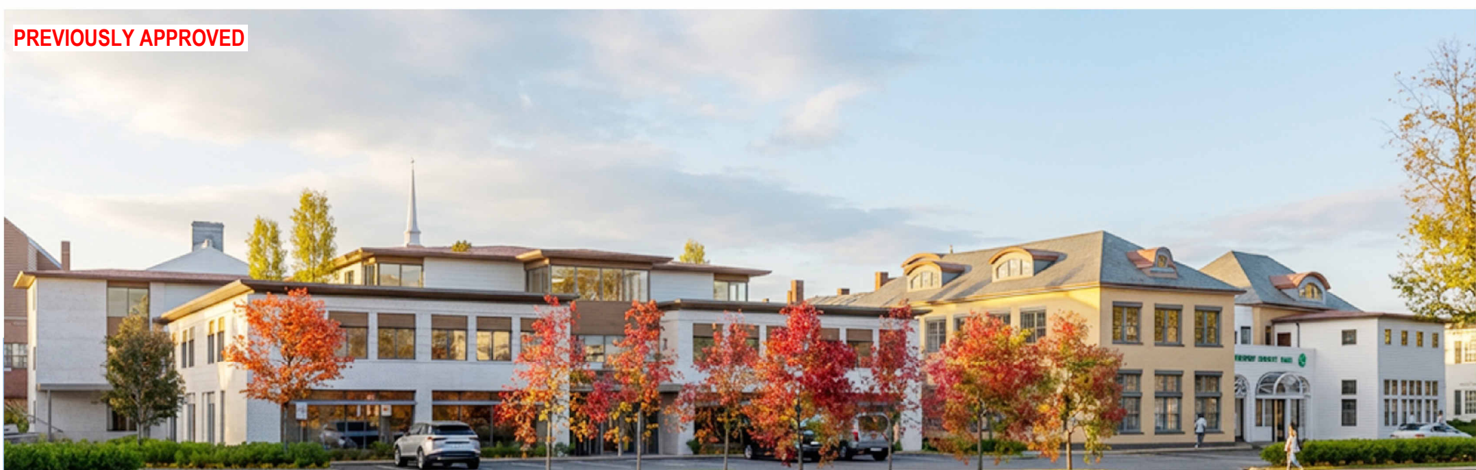
PREVIOUSLY PRESENTED - VIEW FROM SOUTH AT COURTHOUSE
