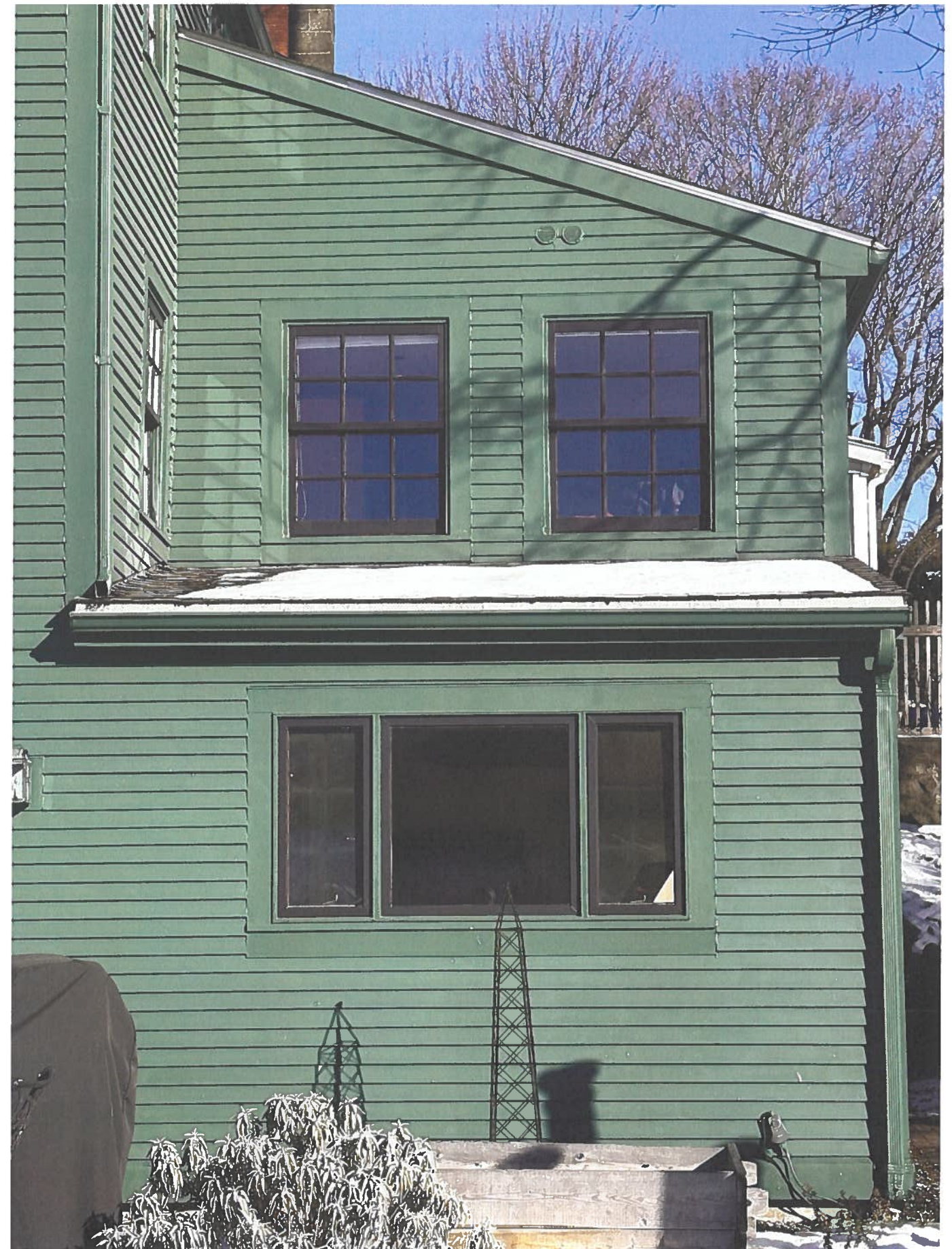
South Elevation: close-up of existing one-story addition
