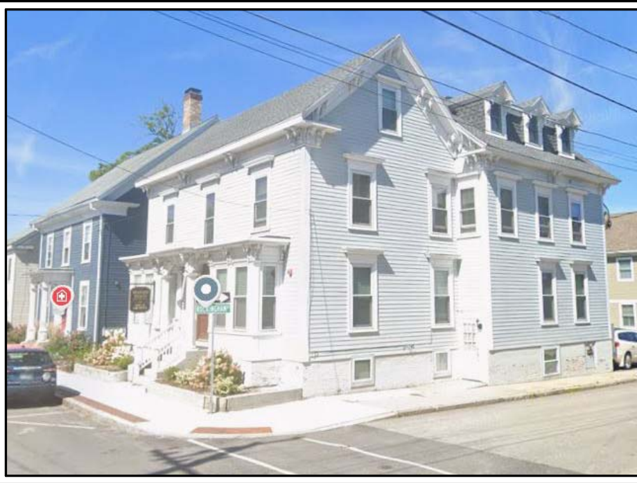
303 ISLINGTON FROM ISLINGTON AND ROCKINGHAM STREET
