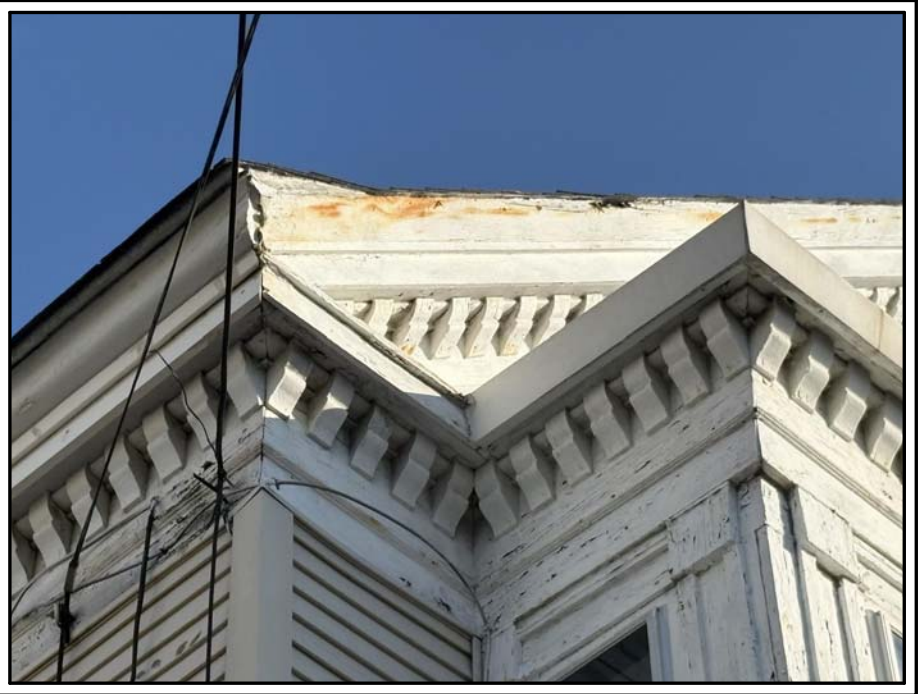
VIEW OF MOLDING, FASCIA, AND TRIM
