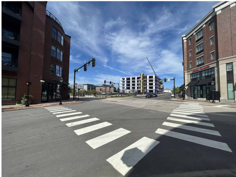
75 DEER ST (IN CONSTRUCTION), 70 MAPLEWOOD AVE, & 162 DEER ST
