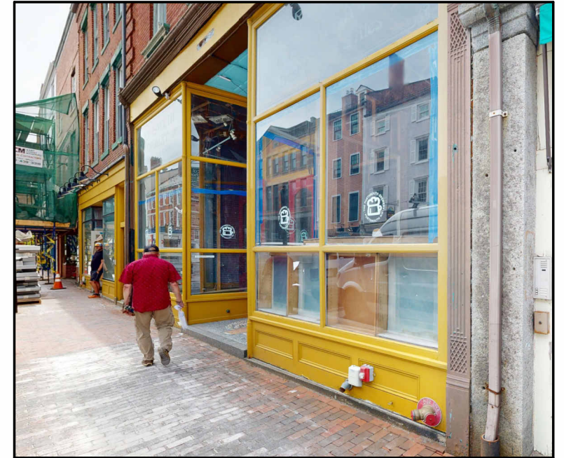
EXISTING STOREFRONT LOOKING SOUTHWEST
