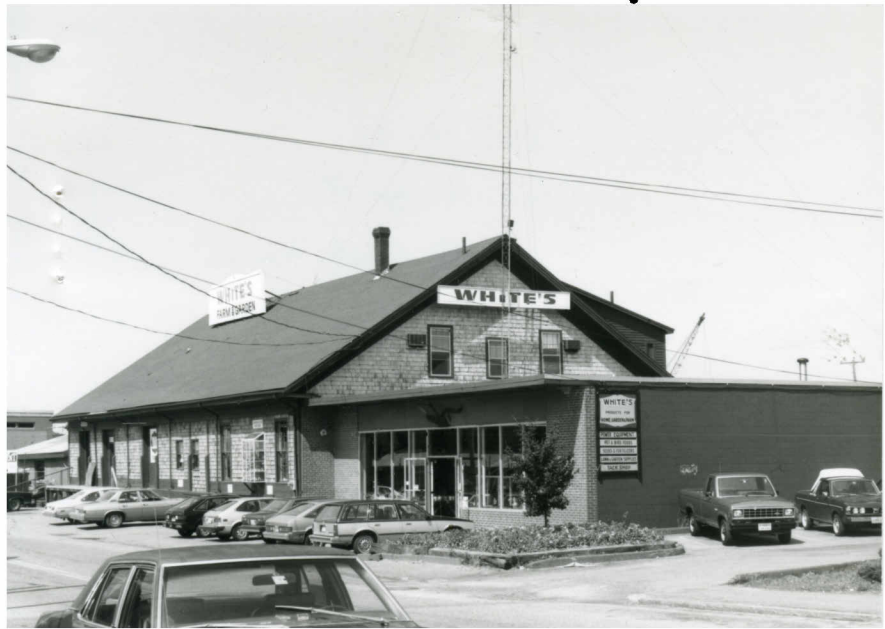
1982 GARDEN SUPPLY PREVIOUS FREIGHT DEPOT
