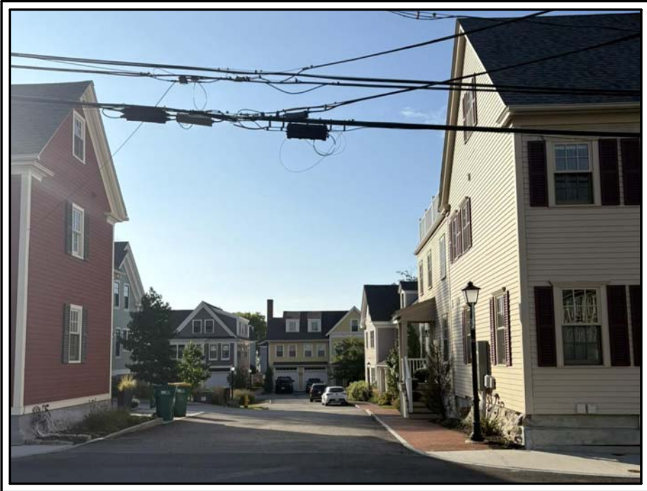
420-430 ISLINGTON ACROSS ISLINGTON STREET
