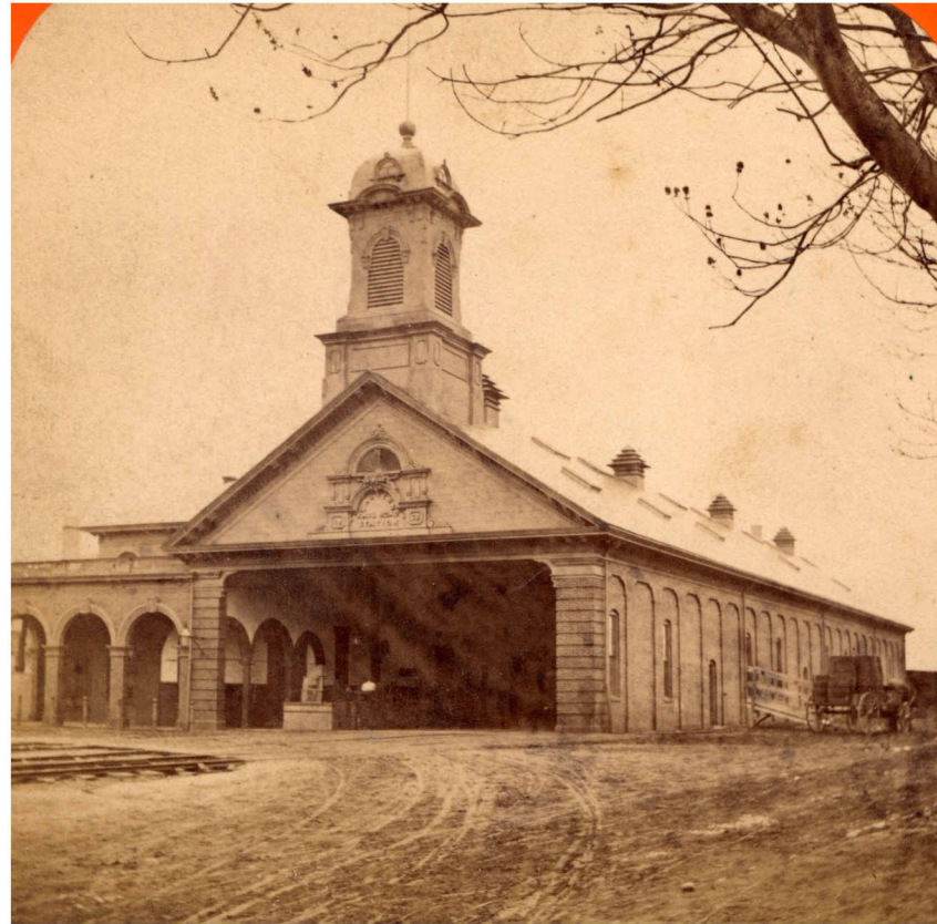
BOSTON & MAINE RAILROAD DEPOT 1864
