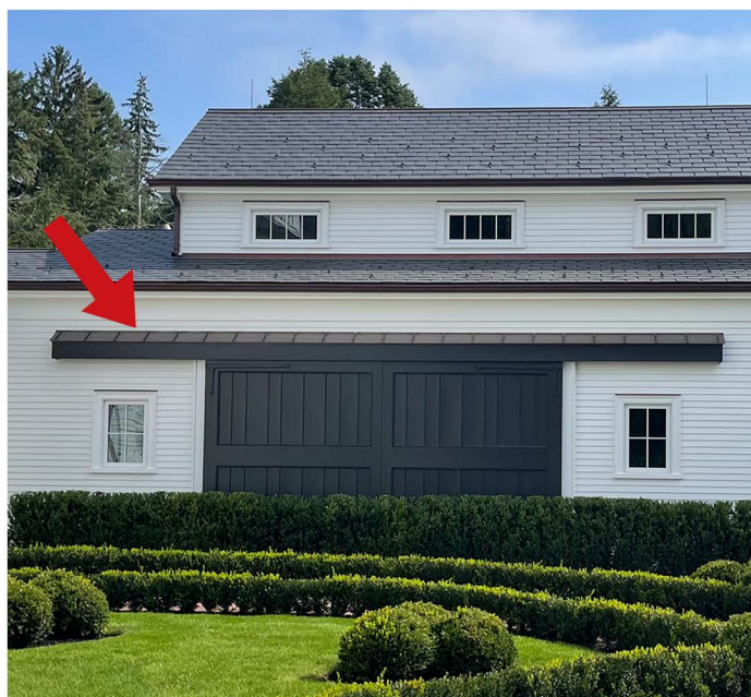
AS-BUILT COPPER ROOF AT FRONT ELEVATION
