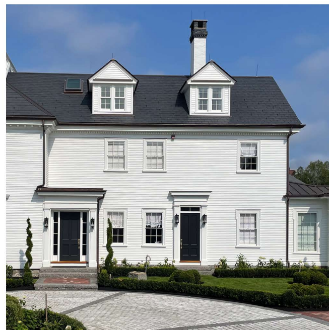
AS-BUILT SOUTH ELEVATION WITH SIX ORIGINAL RESTORED WINDOWS INSTALLED
