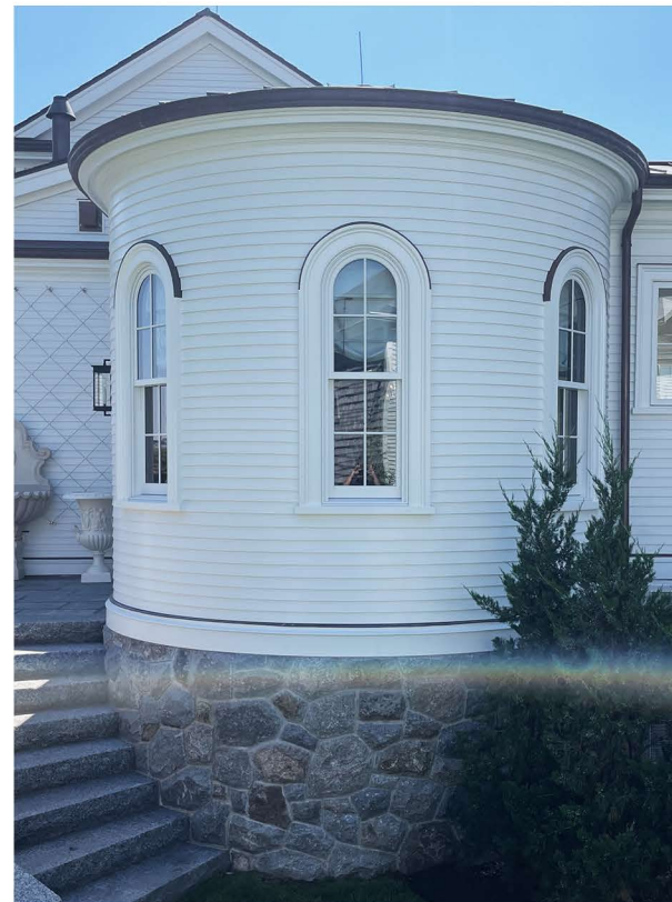
① AS-BUILT CARRIAGE HOUSE SINGLE-HUNG WINDOWS
