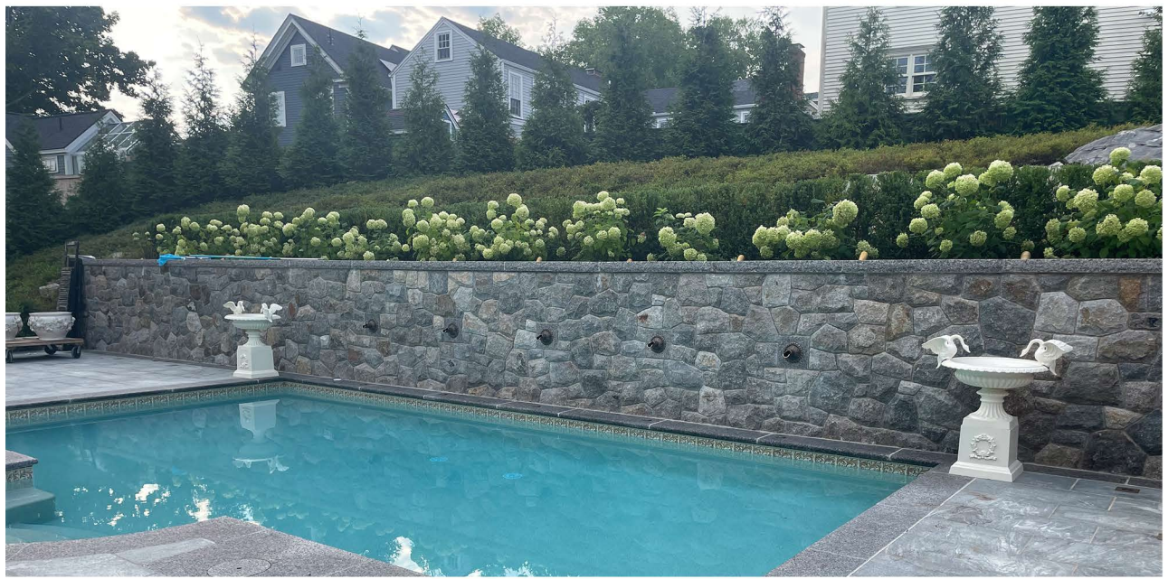
AS-BUILT HILLSIDE RETAINING WALL AT AREA 5
