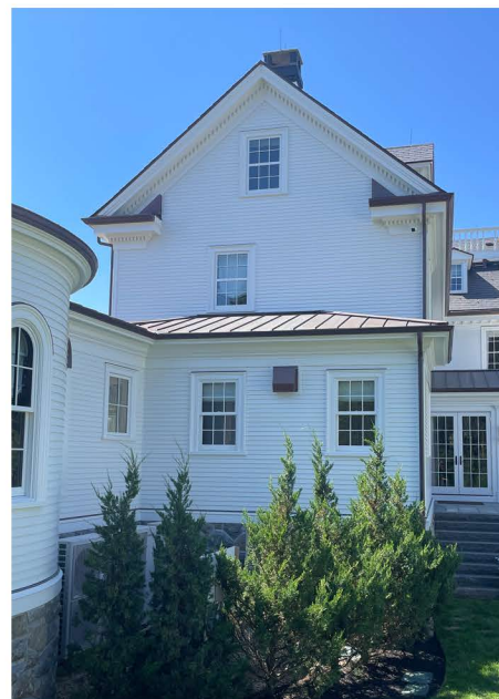
AS-BUILT EAST ELEVATION WITH TWO NEW AND TWO NEW EGRESS CASEMENTS WITH FAUX CHECK FOR EGRESS
