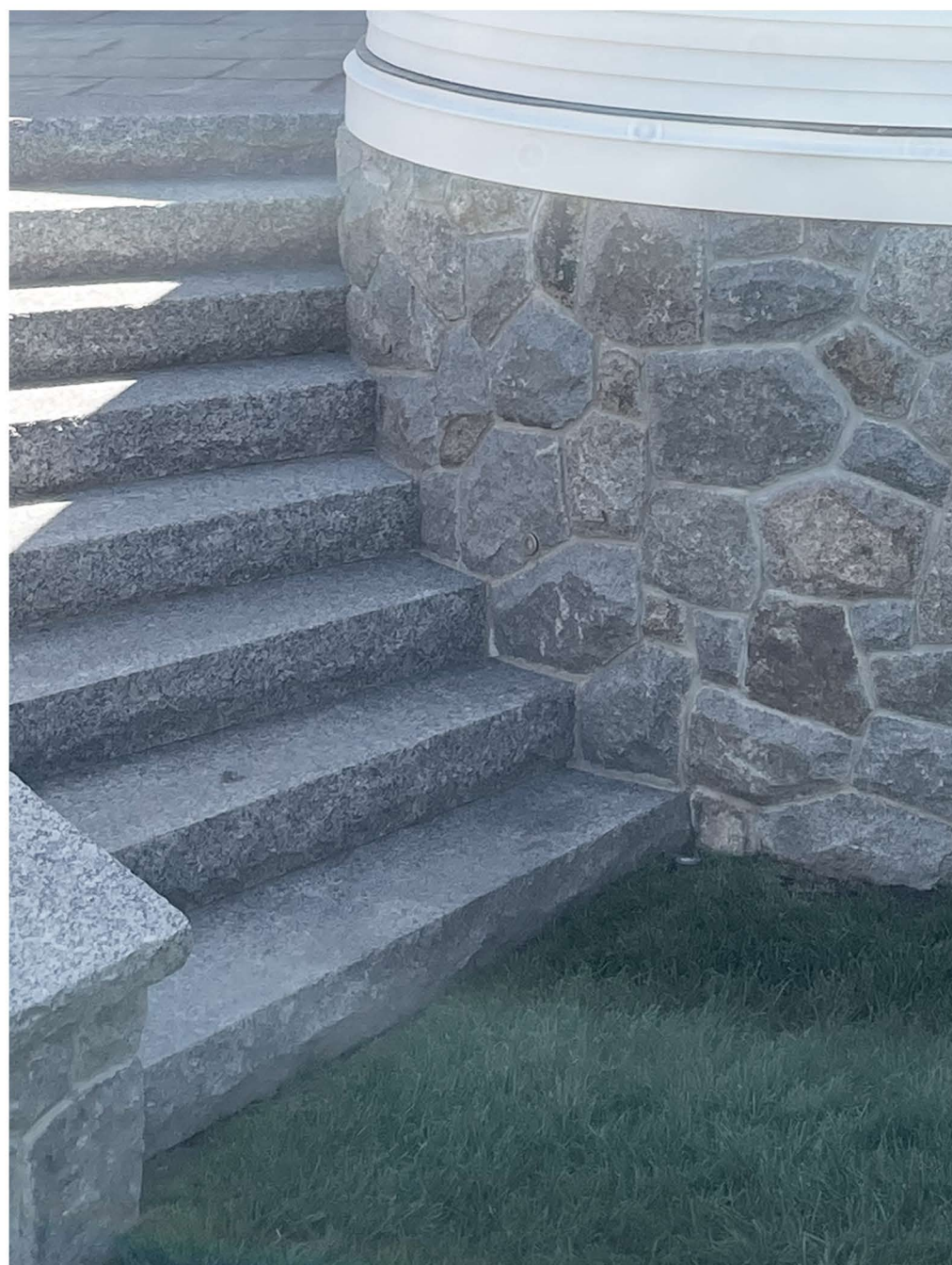
① AS-BUILT APPROVED SQUARE NOSING GRANITE STEPS
