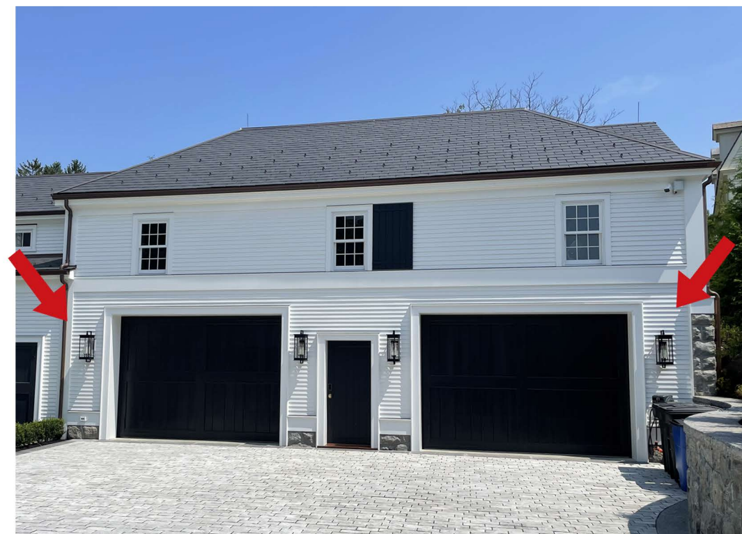
AS-BUILT EXTERIOR LIGHTING AT FRONT ELEVATION
