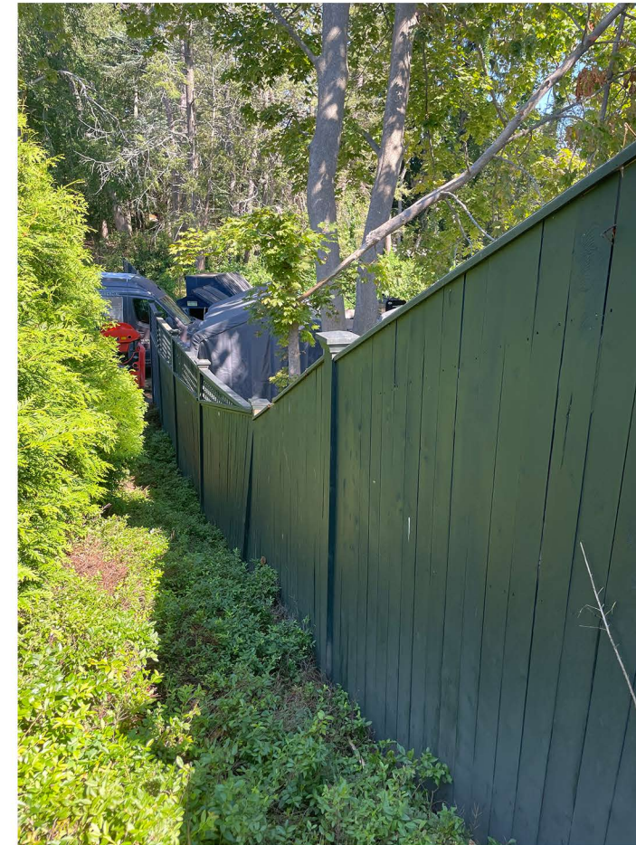
EXISTING FENCE REMAINS NO NEW FENCE INSTALLED AT AREA 2C
