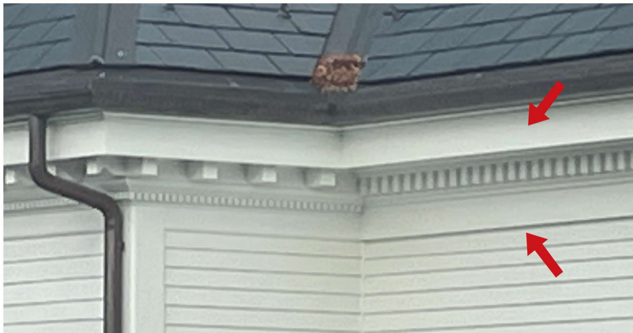
① VIEW OF AS-BUILT CORNICE INTERSECTION
