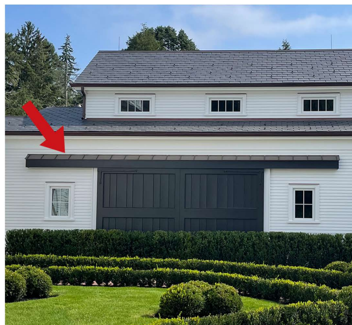
AS-BUILT COPPER ROOF AT FRONT ELEVATION
