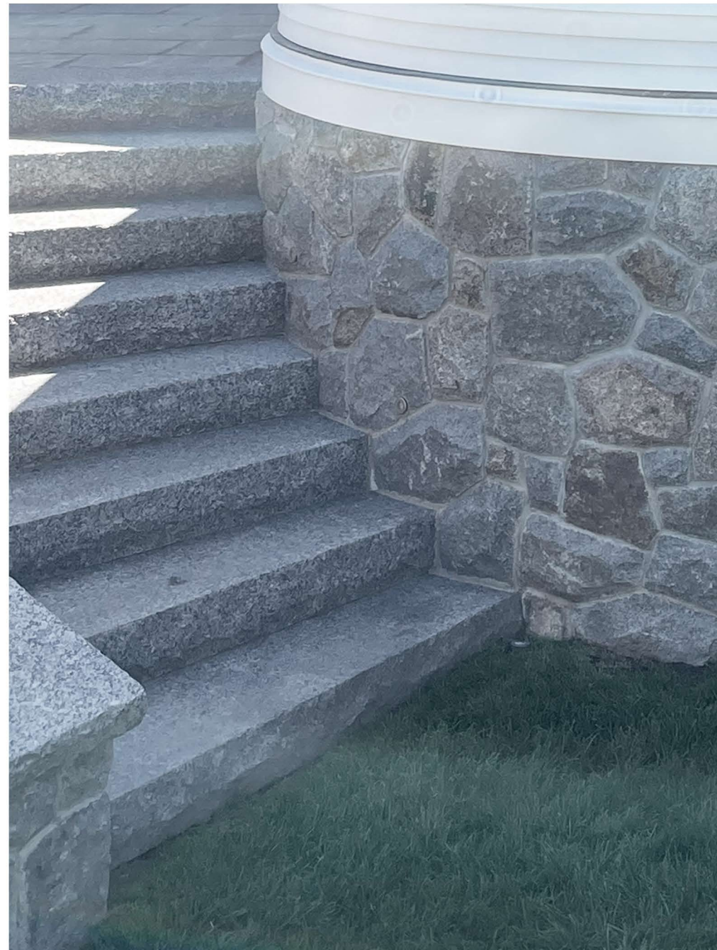
① AS-BUILT APPROVED SQUARE NOSING GRANITE STEPS
