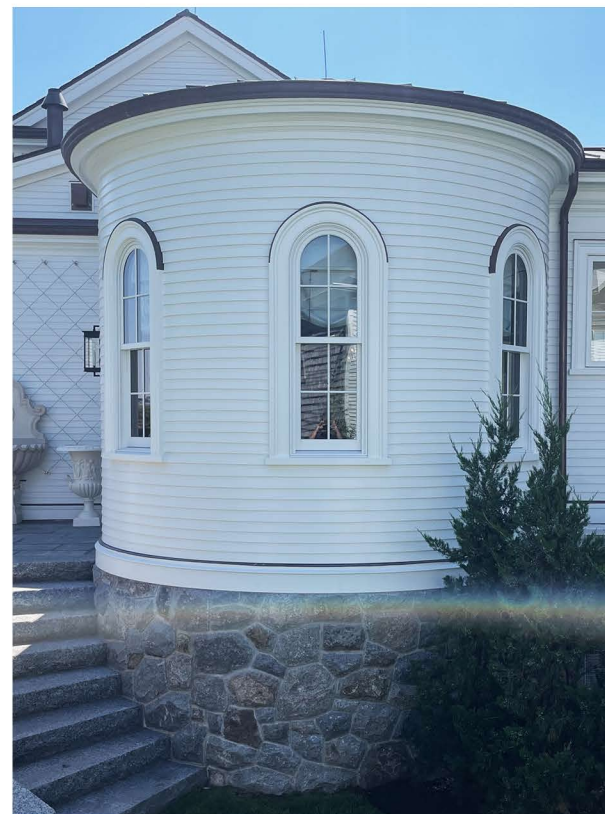
① AS-BUILT CARRIAGE HOUSE SINGLE-HUNG WINDOWS
