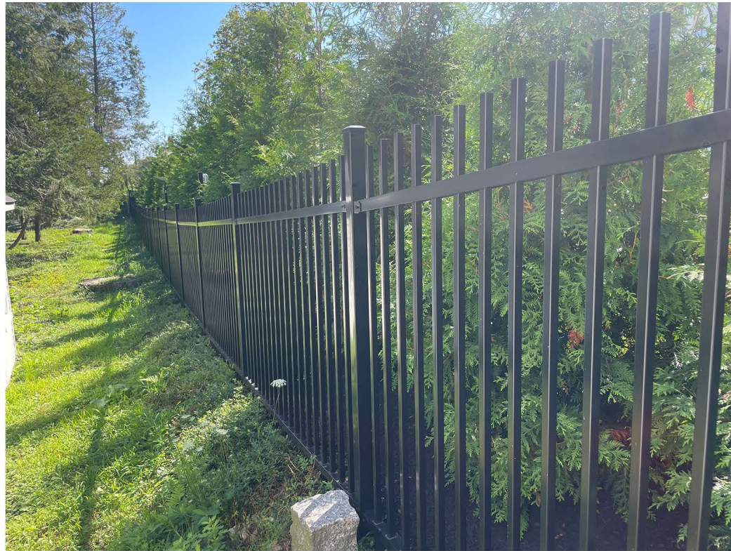
VIEW OF AS-BUILT ALUMINUM FENCE
