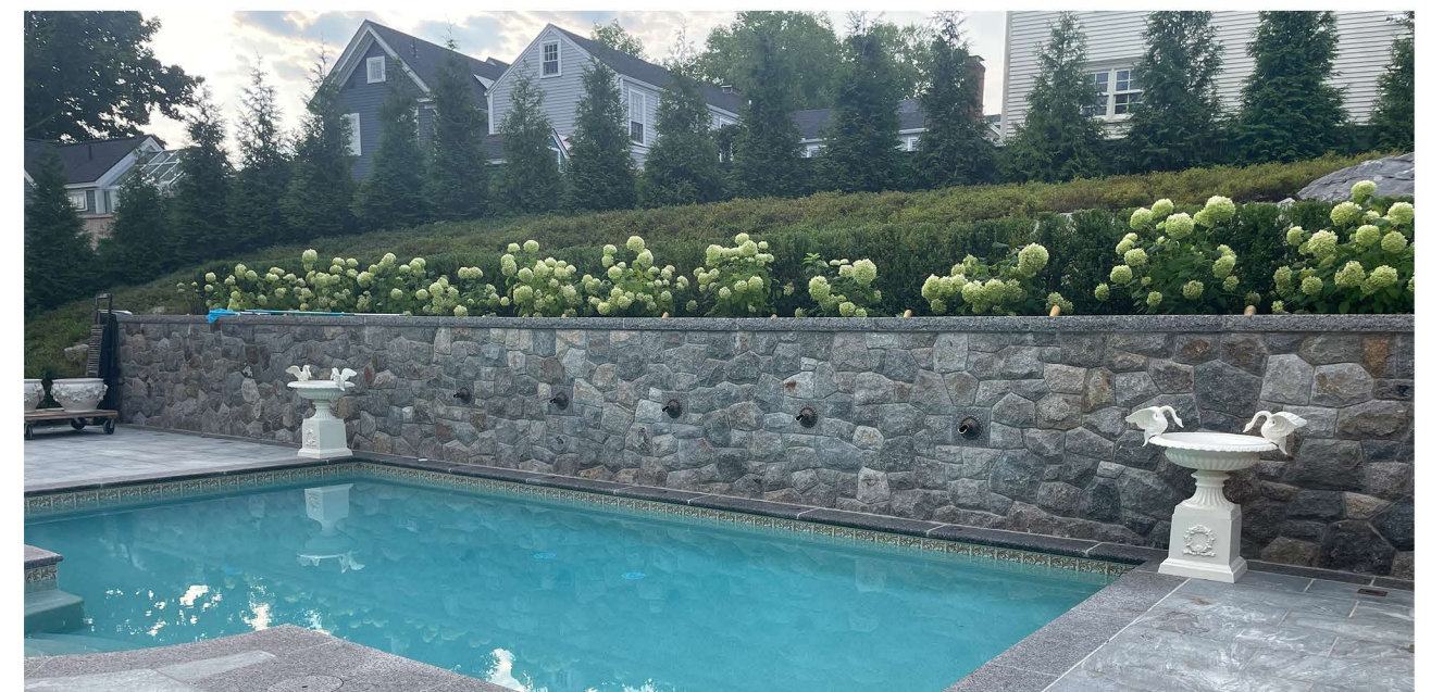
AS-BUILT HILLSIDE RETAINING WALL AT AREA 5
