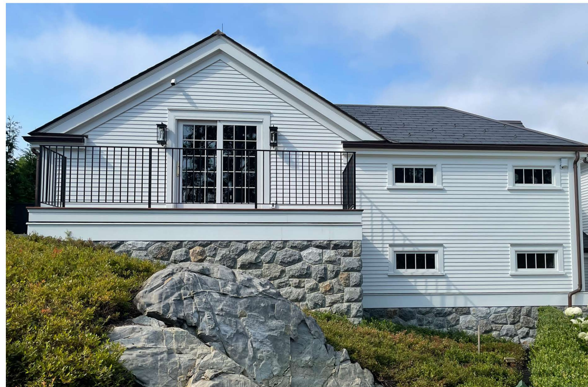
② AS-BUILT PHOTO OF CARRIAGE HOUSE REAR ELEVATION
