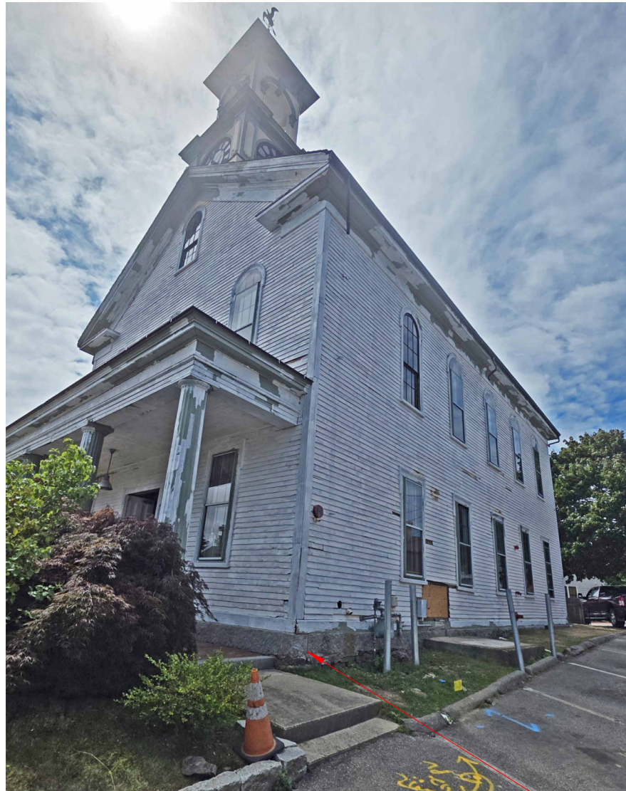
NORTHEAST GRANITE SILL REPLACEMENT
