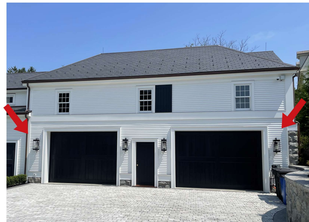
AS-BUILT EXTERIOR LIGHTING AT FRONT ELEVATION
