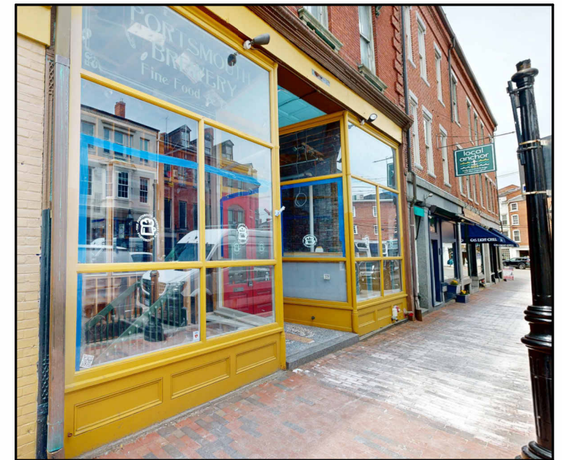
EXISTING STOREFRONT LOOKING NORTH WEST
