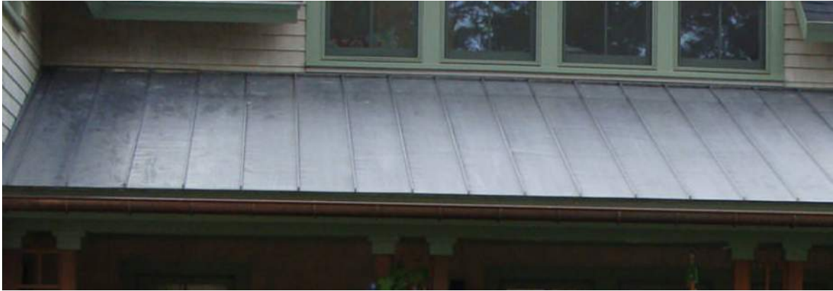
STANDING SEAM LEAD COATED COPPER ROOF
