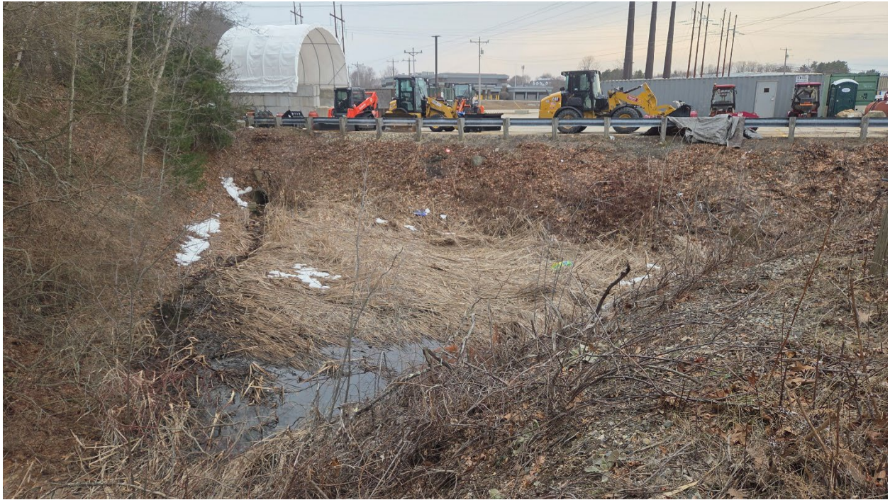
Photo 11 – Liberty Mutual – View looking west within the Stormwater Area and towards the outlet of Culvert $4 (Photo taken 3/20/2026).
