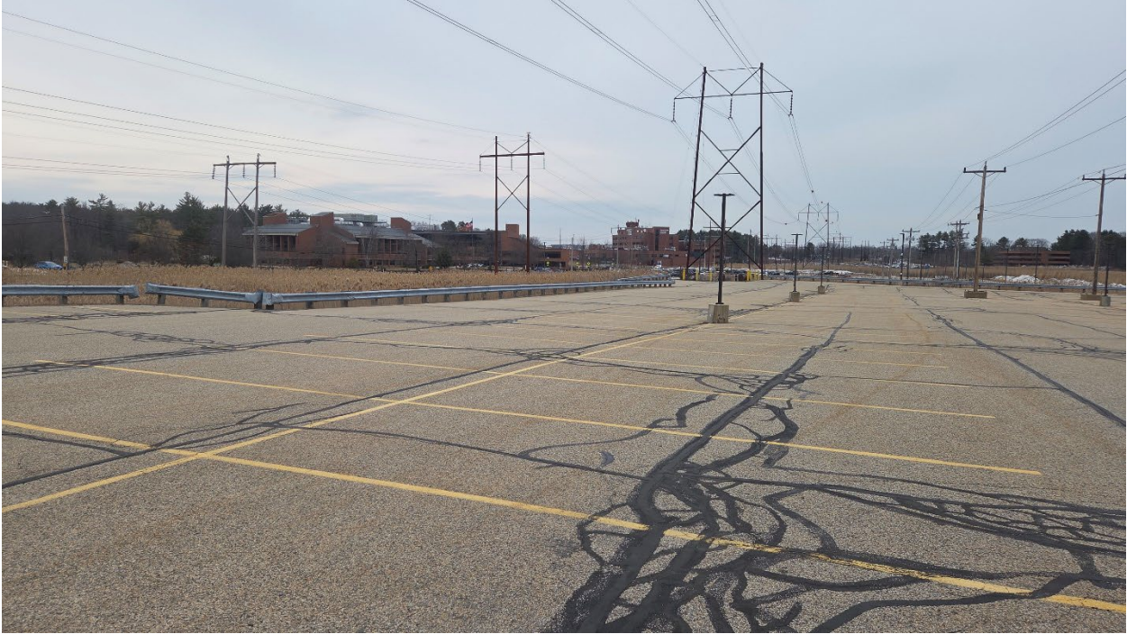
Photo 1 – Liberty Mutual – View looking east along the parking lot which drains toward the Stormwater Area (Photo taken 3/20/2026).
