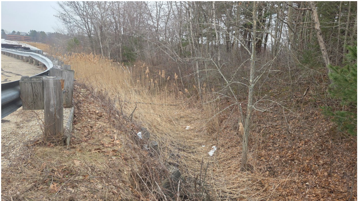
Photo 10 – Liberty Mutual – View looking along the Stormwater Area (Photo taken 3/20/2026).
