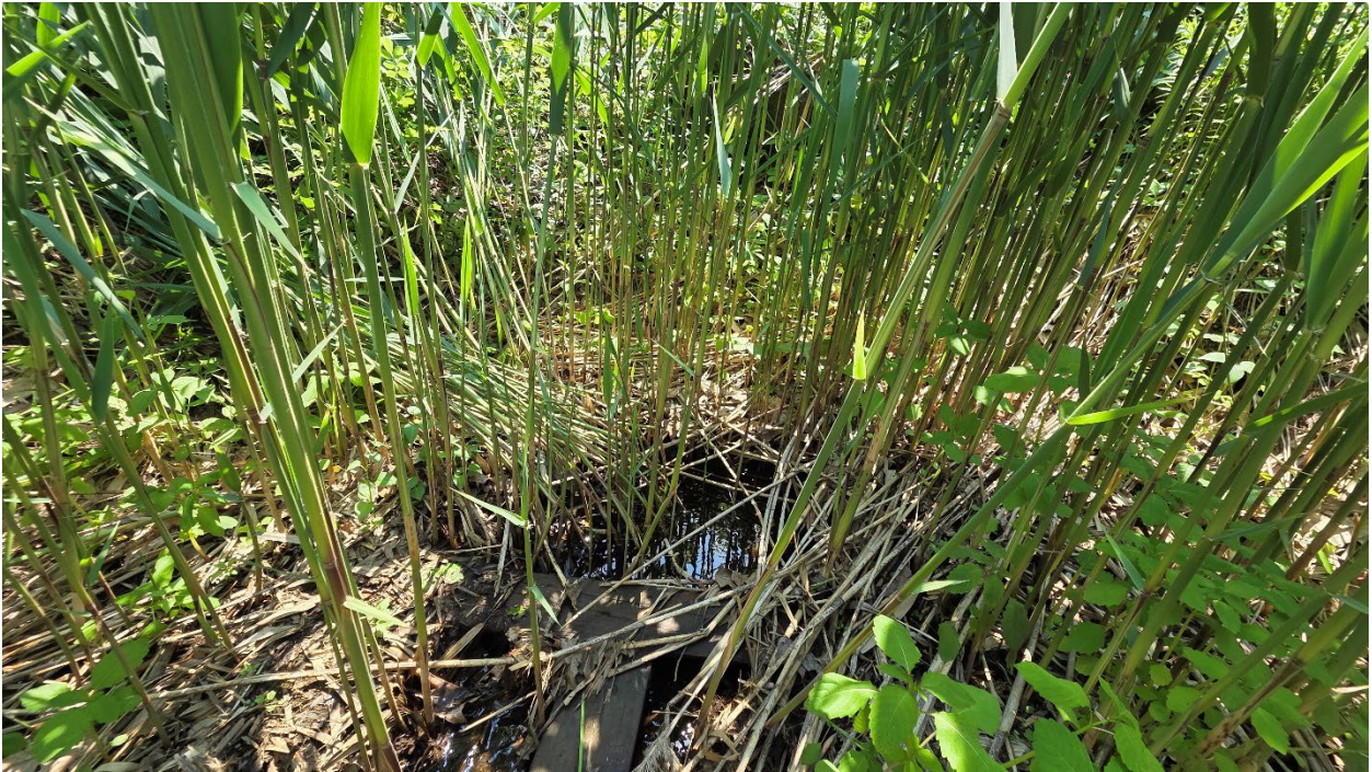
Photo 14 – Liberty Mutual – View of the outlet of Culvert #1 (Photo taken 6/5/2025)
