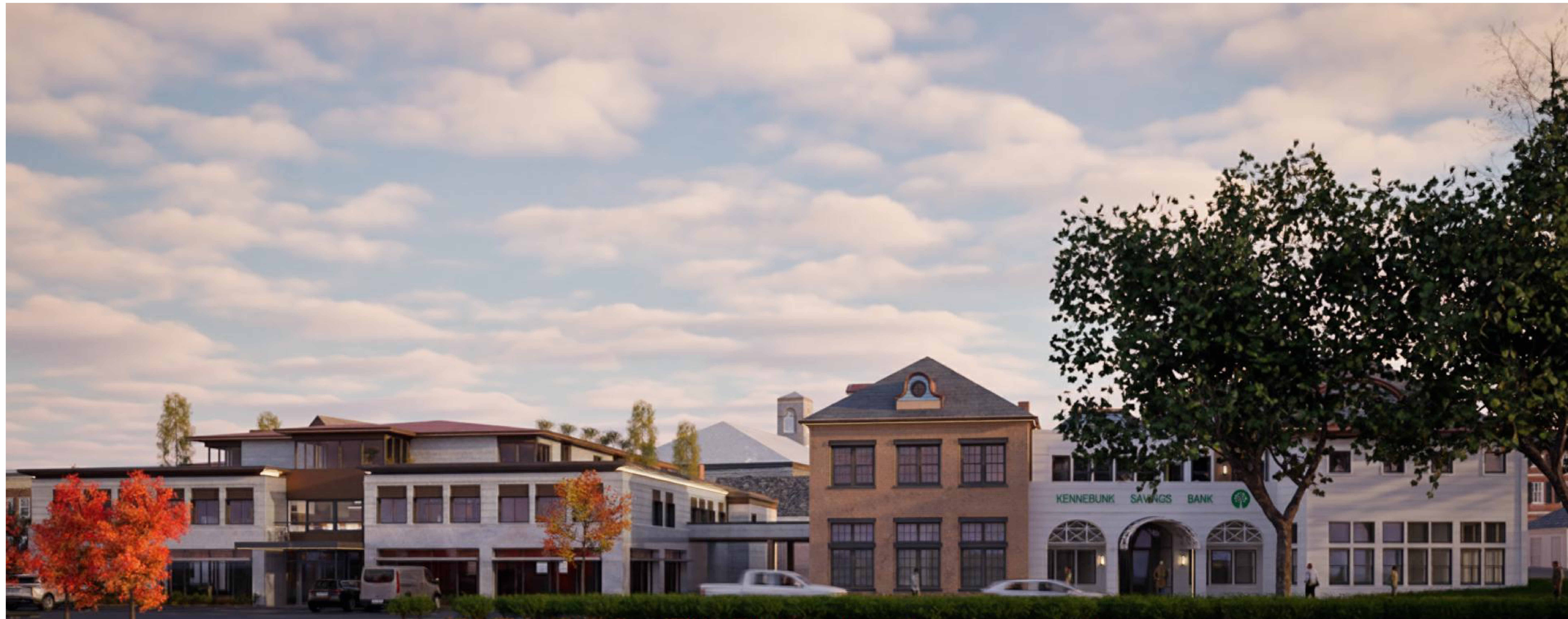
VIEW FROM JUNKINS AVENUE AT CITY HALL PB
