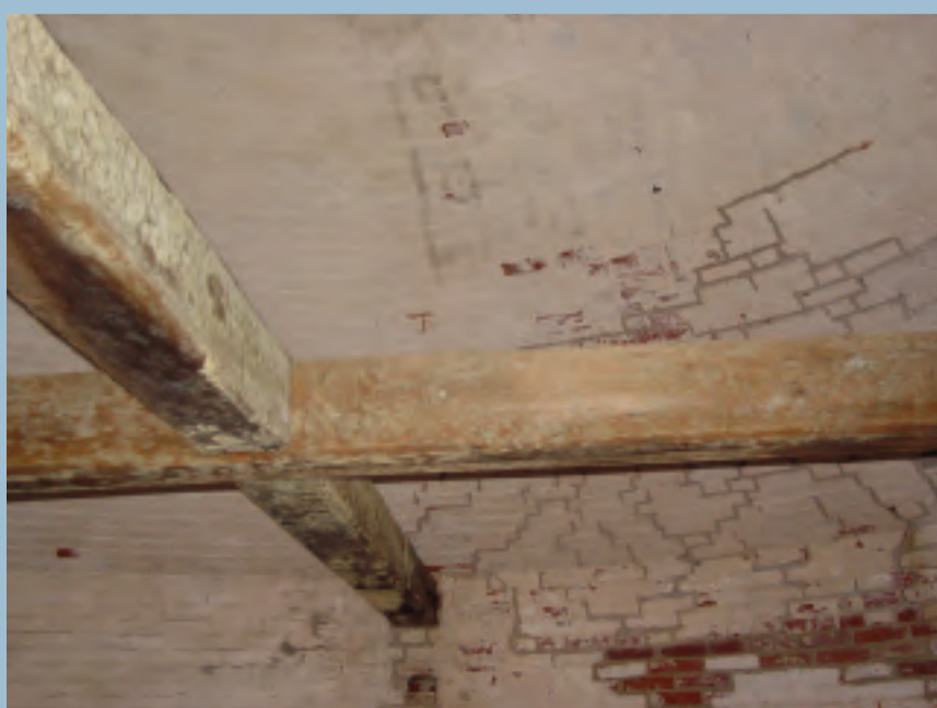
Photograph of wooden beams on ceiling. Courtesy of City of Portsmouth.
