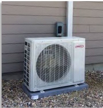
Heat pump (Mini-Split System)
