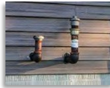
Oil tank pipes
