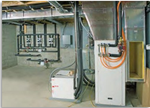
Geo-Thermal System in basement
