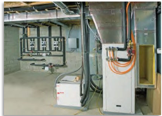
Geo-Thermal System in basement
