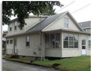
EAF/BAS/UBM Attic + dormer
