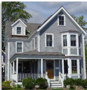
EAF/FUS/BAS/UBM Attic + turns in roof
