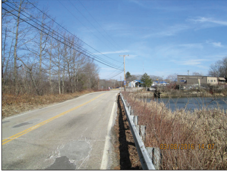
PHOTO 9 - BANFIELD RD AT APPROX STA 192+00 LOOKING NORTH AT PEVERLY HILL ROAD
