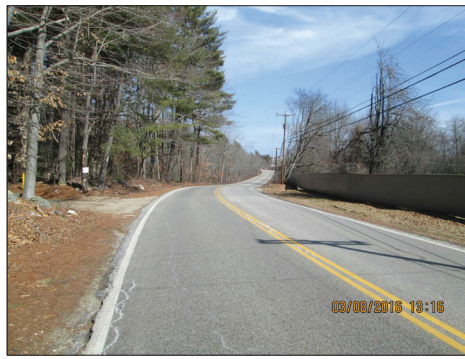
PHOTO 7 - BANFIELD RD AT APPROX STA 165+00 LOOKING NORTH
