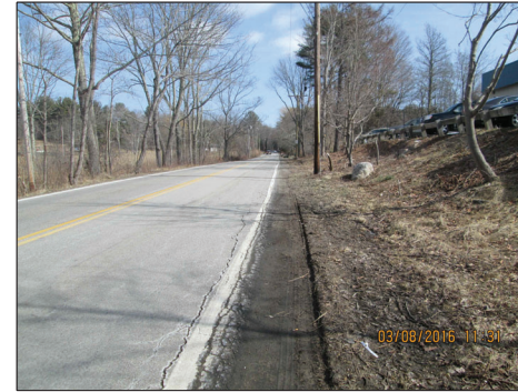
PHOTO 3 - BANFIELD RD AT APPROX STA130+00 LOOKING NORTH
