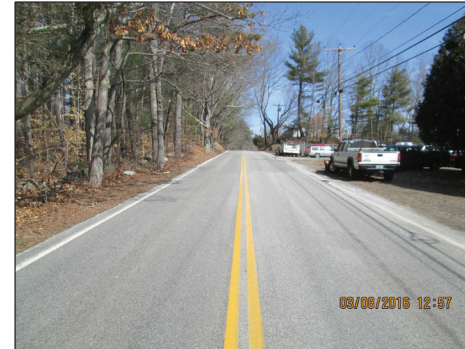
PHOTO 5 - BANFIELD RD AT APPROX STA 158+00 LOOKING NORTH
