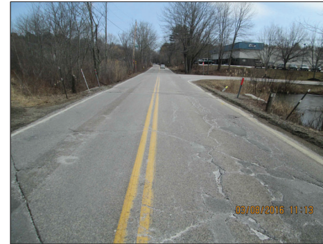
PHOTO 2 - BANFIELD RD AT APPROX STA 126+00 (BAN-4) LOOKING NORTH
