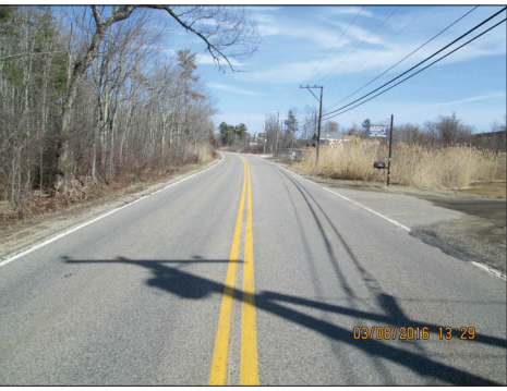
PHOTO 8 - BANFIELD RD AT APPROX STA 171+00 LOOKING NORTH
