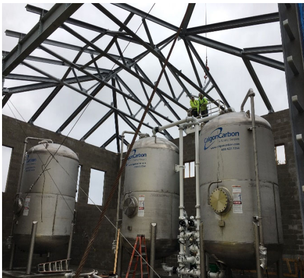
Installation of New Carbon Filters
