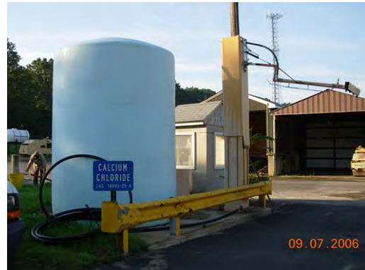
Figure 38. Overhead Pre-Wet Spray System
