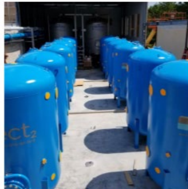
IOX Resin Filter Vessels
