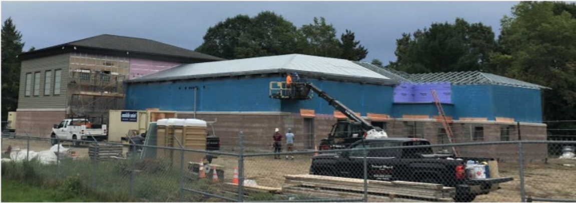
Construction of New Drinking Water Treatment Facility Upgrade – October 2020
