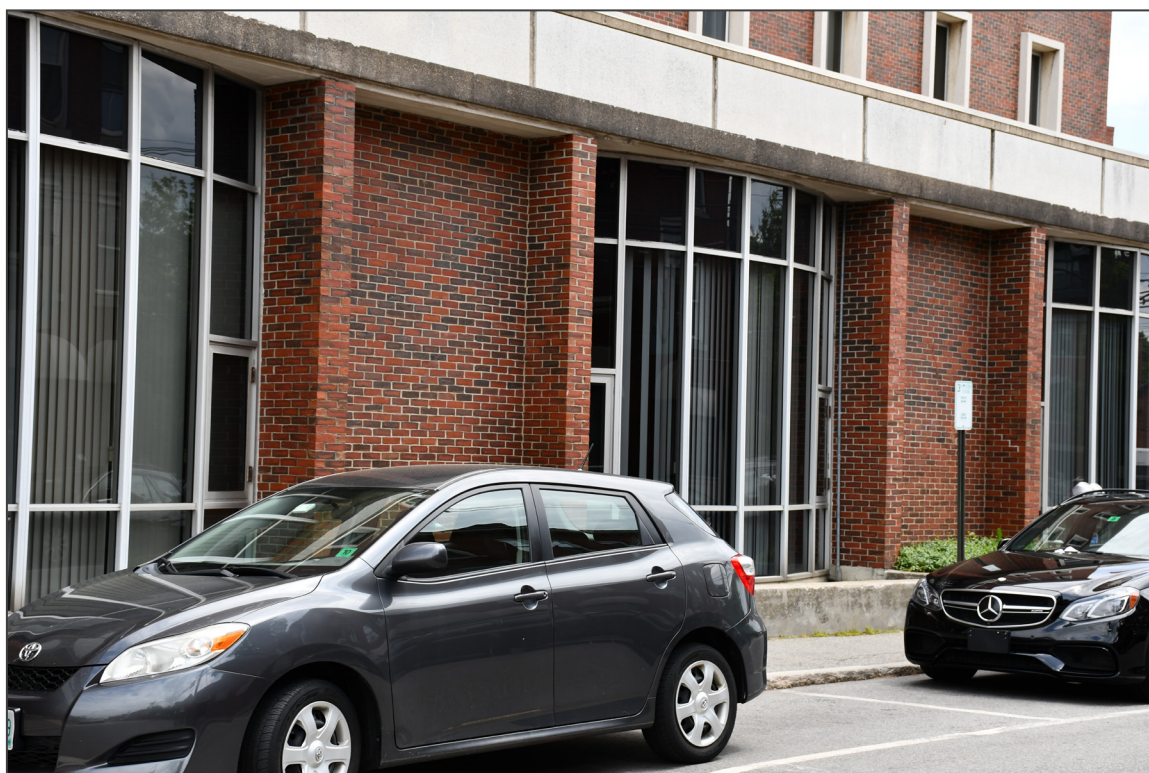
22. West elevation, facing southeast
