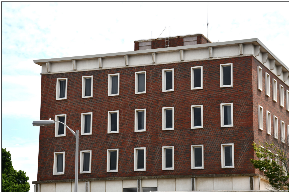
18. North elevation, facing southeast
