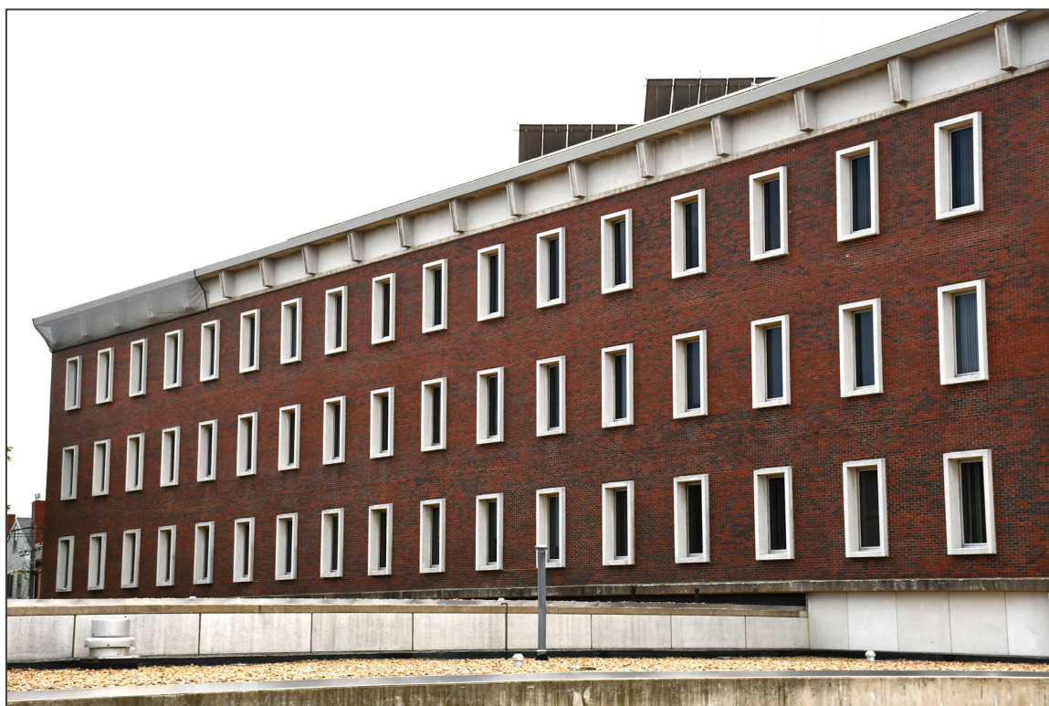
14. East elevation, facing southwest
