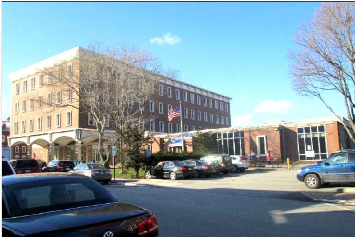
9. South and east elevations, facing northwest
