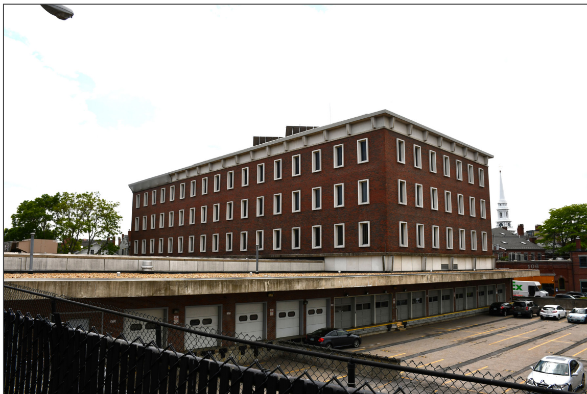
13. East and north elevations, facing southwest
