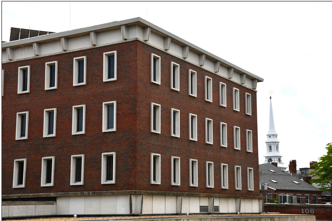
15. East and north elevations, facing southwest
