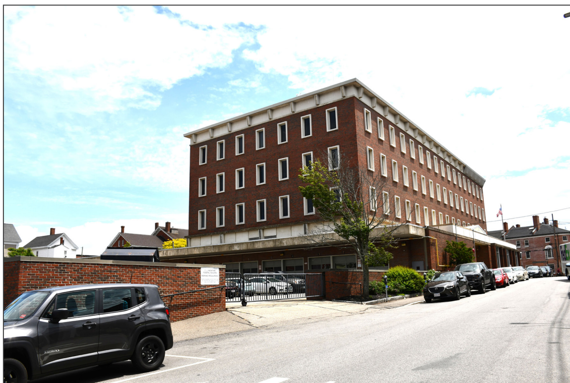
20. North and west elevations, facing southeast
