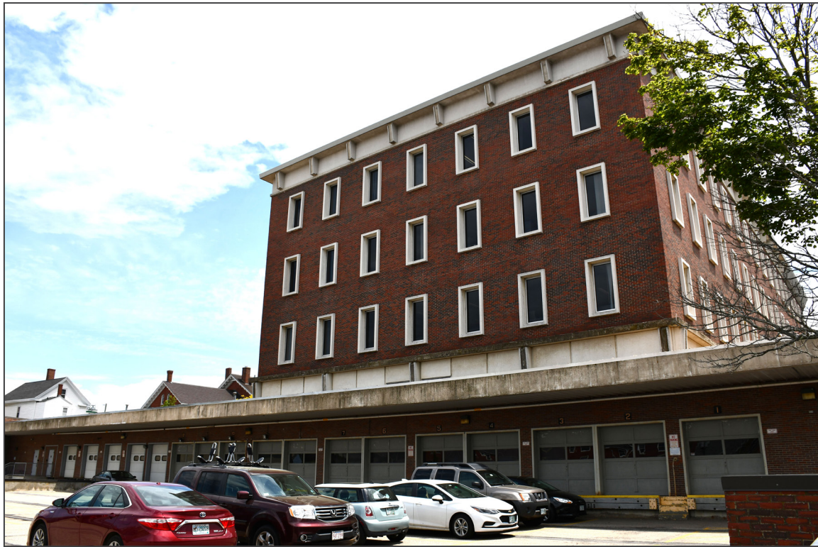
17. North elevation, facing southeast
