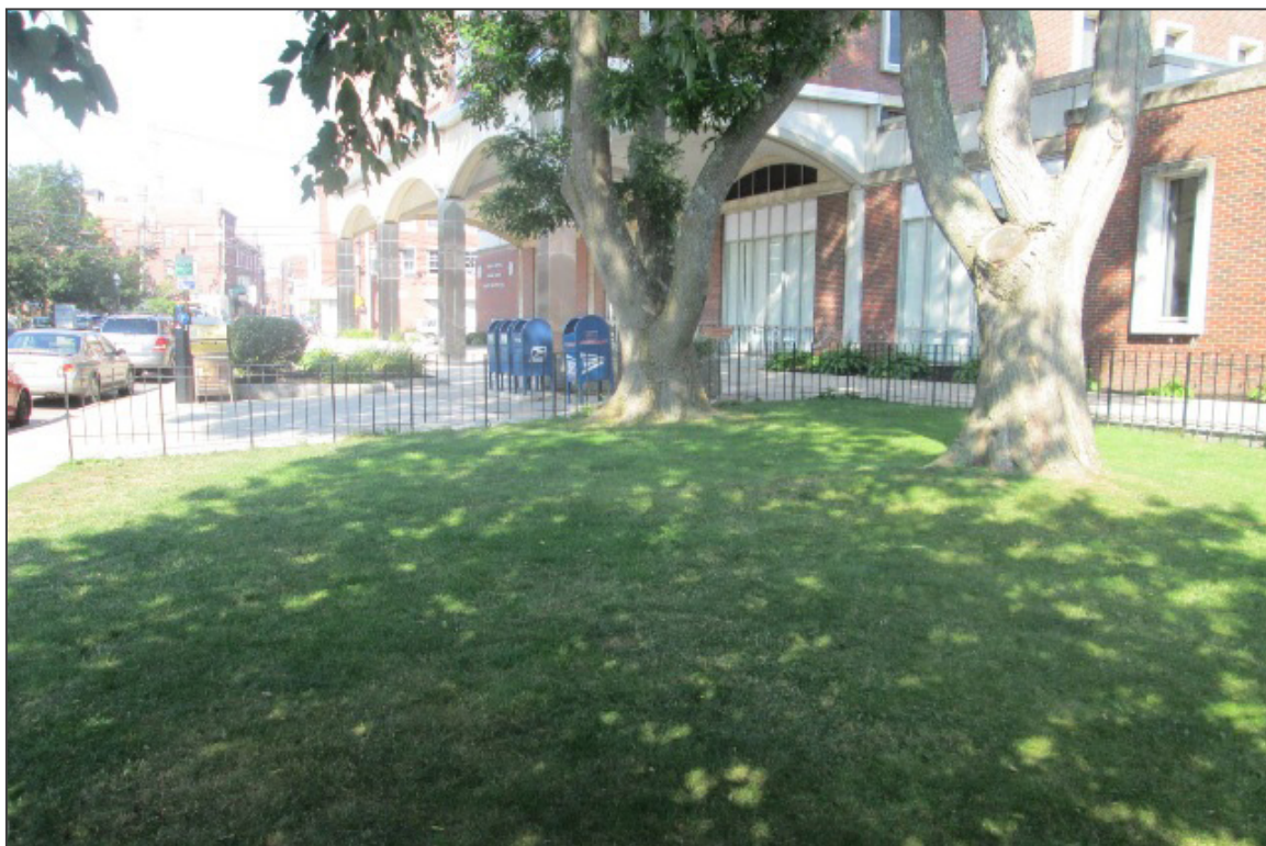
10. Site and south elevation, facing northwest
