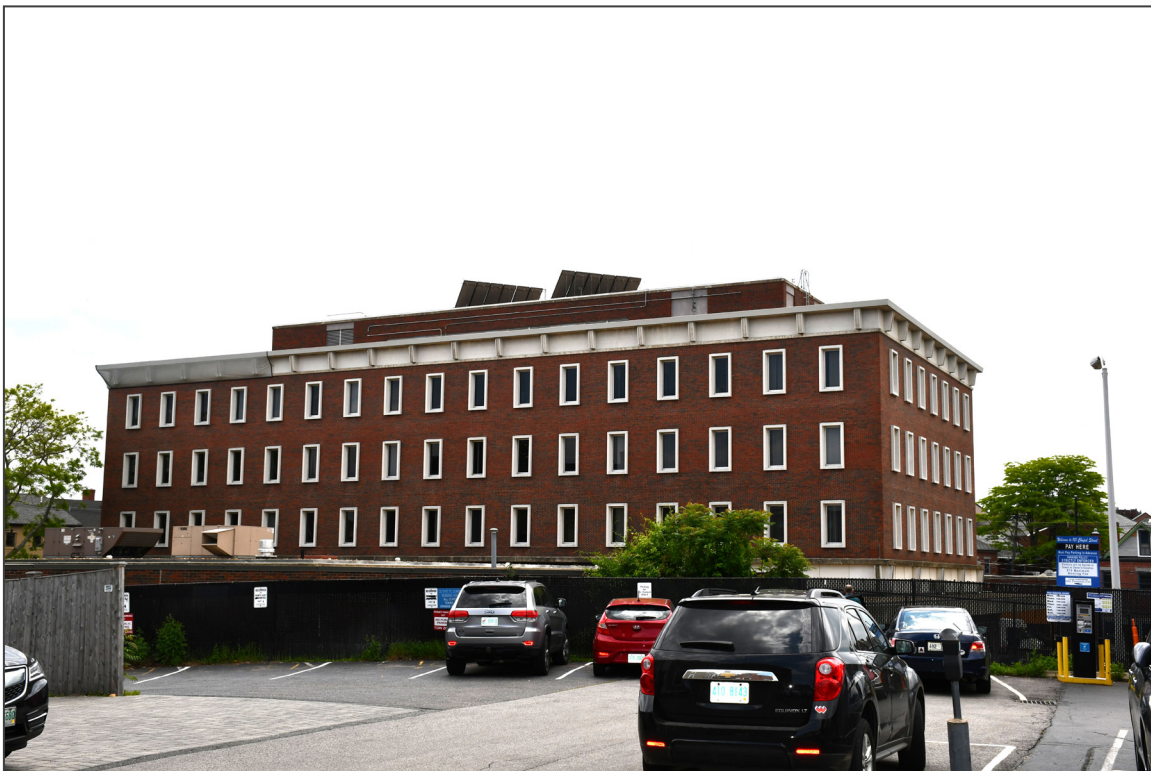
12. East and north elevations, facing southwest
