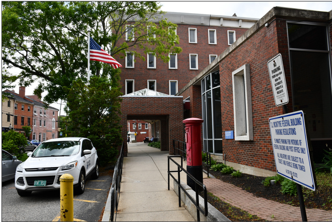
7. East and south elevations, facing west
