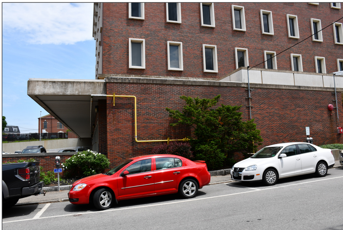
21. West elevation, facing southeast
