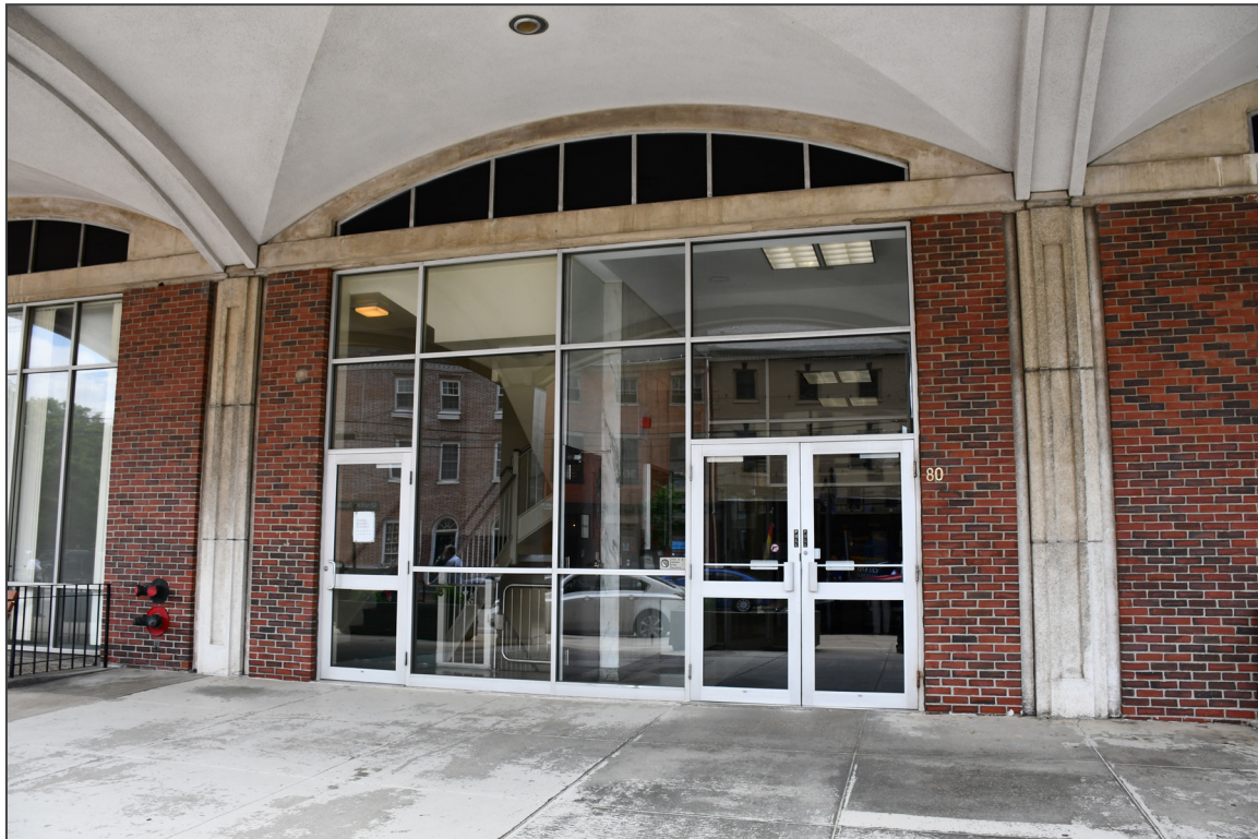
3. South elevation, facing north
