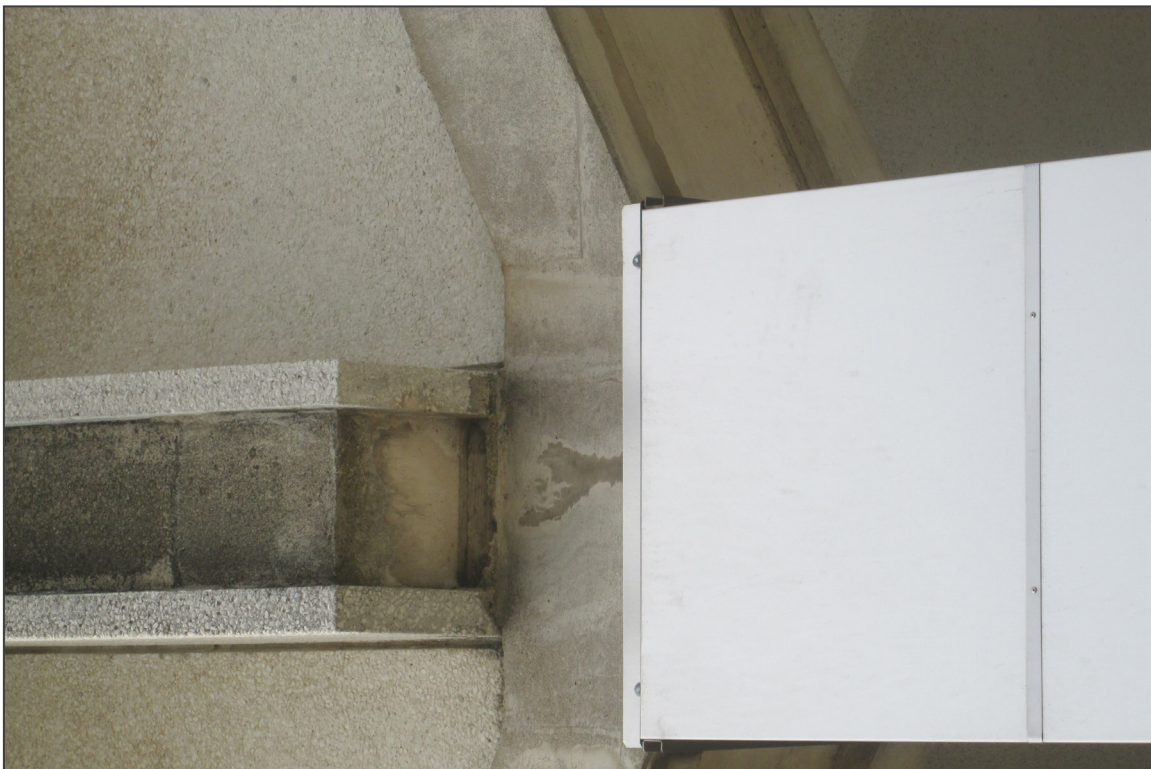
28. South elevation column detail
