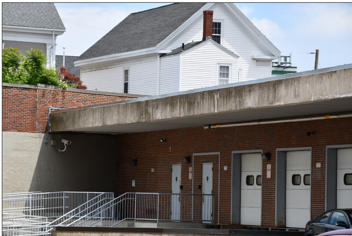
19. North elevation, facing southeast
