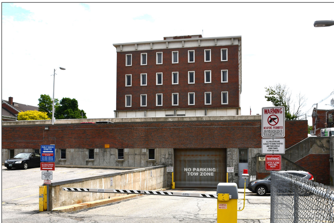
16. North elevation, facing south
