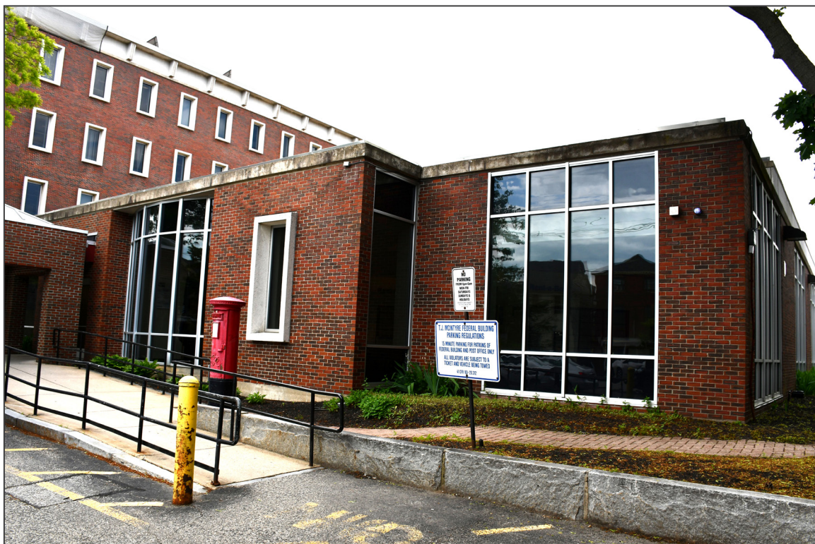
8. East and south elevations, facing northwest
