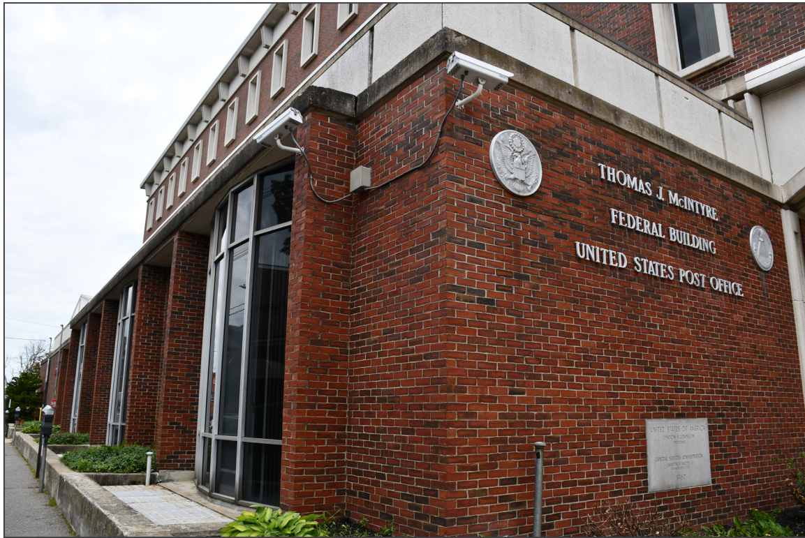
1. West and south elevations, facing northeast
