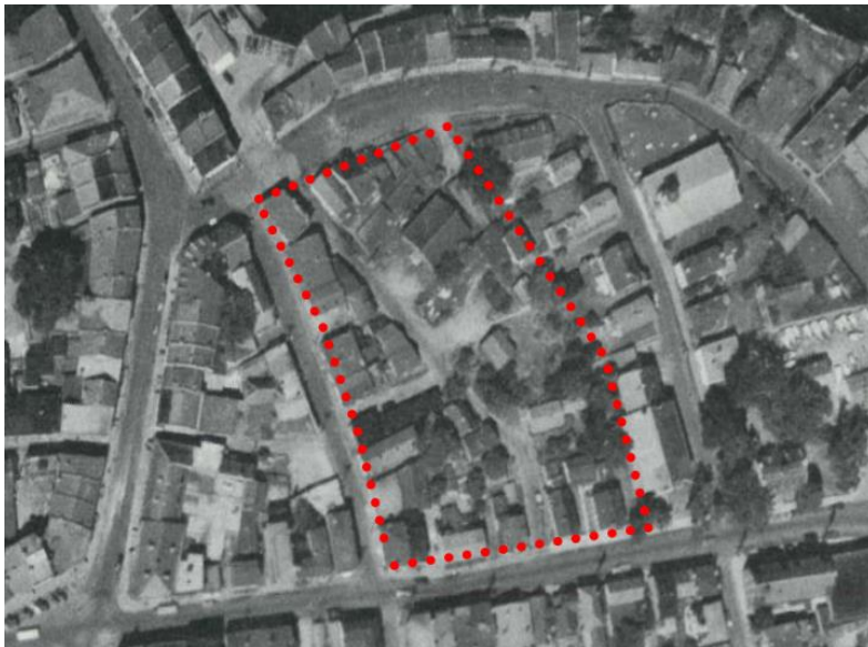
1: Aerial of site prior to McIntyre building construction
