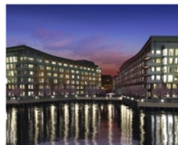
Fairmont Battery Wharf
