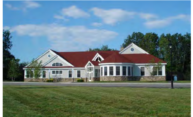
Tighe & Bond 177 Corporate Drive, Portsmouth NH
