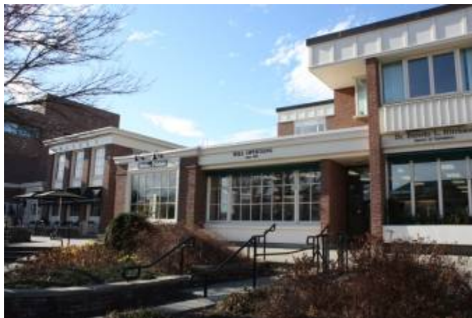
Nugget Building and Hanover Improvement Assoc., Hanover (1951 & 1970)
