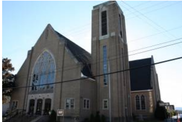
St. George's Church, Manchester (1953 ). Leo Provost, architect
