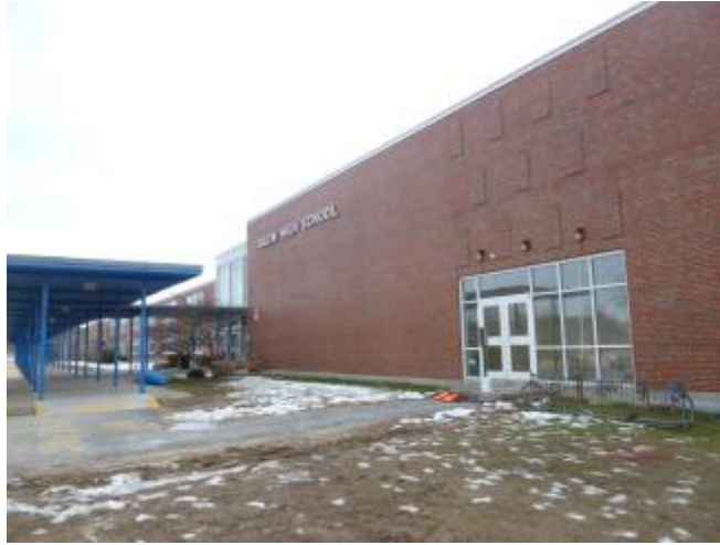
Salem High School, Salem (1968). Irving W. Hersey Associates
