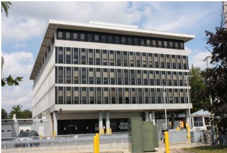
James Cleveland Federal Building, Concord (1966) Koehler & Isaak, architects
