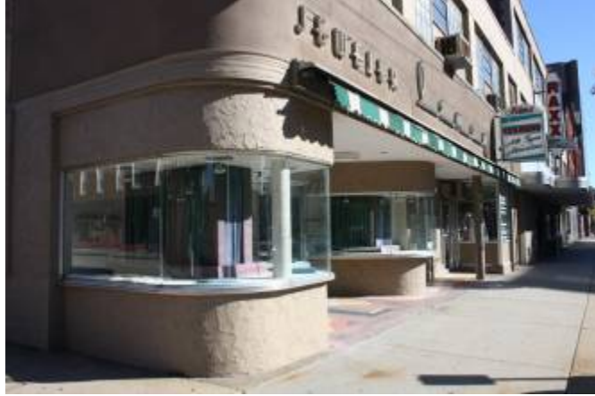
Lee Building, 1-5 N. Main Street, Concord (1957)
