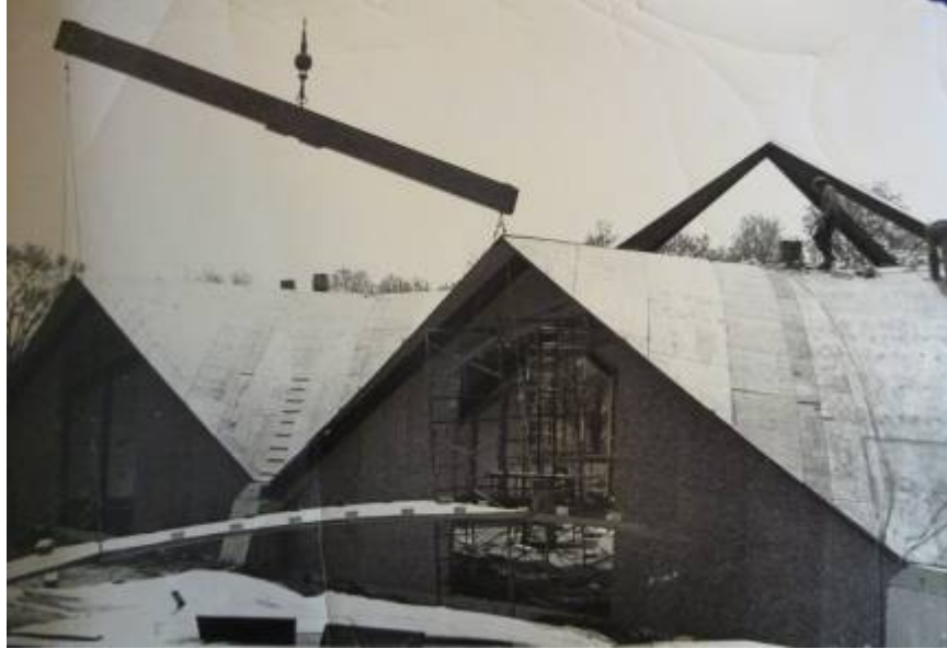
Smart Gymnasium under construction, Spaulding Youth Center, Tilton (1970)
