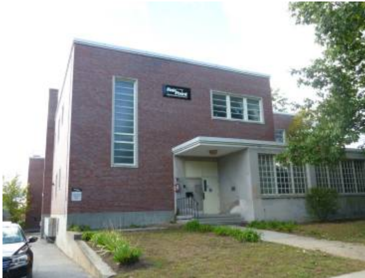
Dial Central Office Building, Keene (1958) Alfred T. Granger Associates, architect
