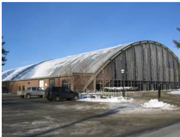
Leverone Field House, Dartmouth College, Hanover (1961-3) Pier Luigi Nervi, architect
