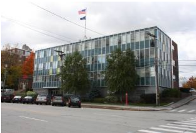
NH Employment Security, Concord (1958). Koehler & Isaak, architects
