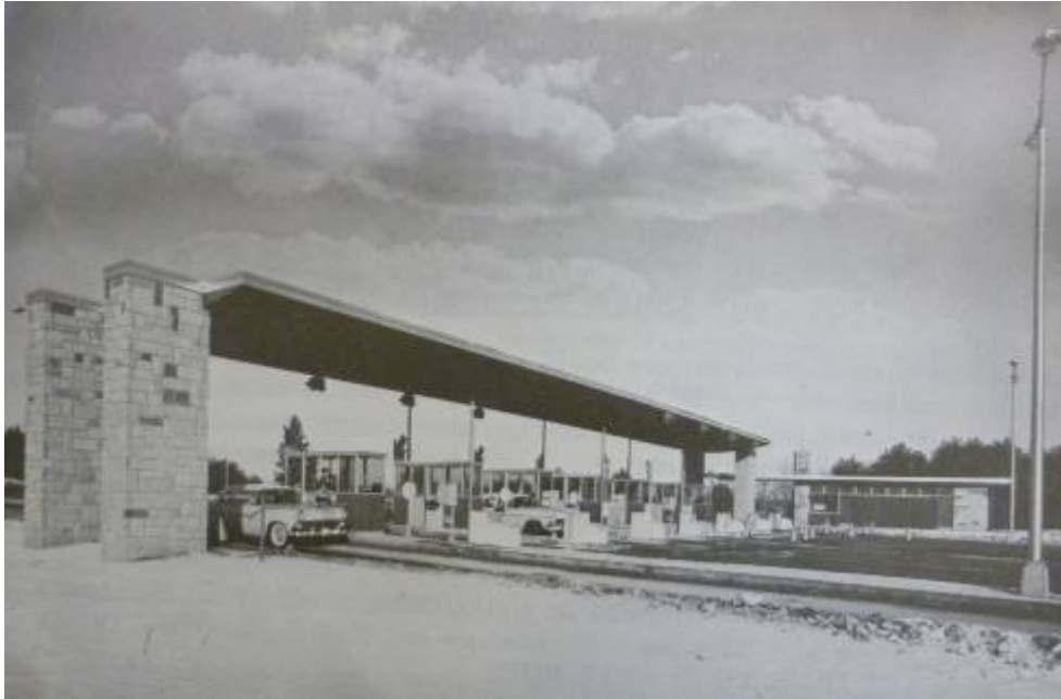
Toll Houses on Everett Turnpike at Merrimack E.H. and M.K. Hunter, architects
