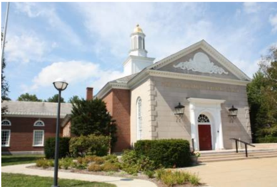
Supreme Court Building, Concord (1969) Royal Barry Wills Associates, architects
