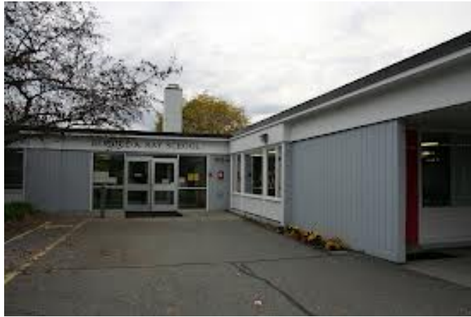
Bernice Ray Elementary School, Hanover (1968). Roy Banwell, architect
