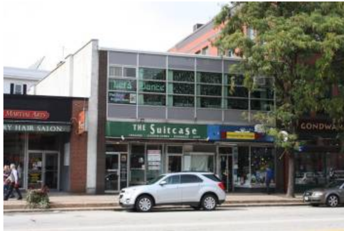
Prescription Center, N. Main Street, Concord (1971). Guy K.C. Wilson, architect
