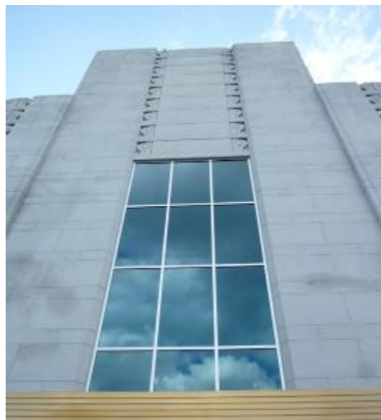
Details, NH Fire Insurance Building, Manchester
