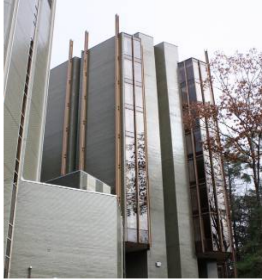
Williamson & Christensen Halls, Philbrook, UNH, Durham (1969-1973). Ulrich Franzen, architect
