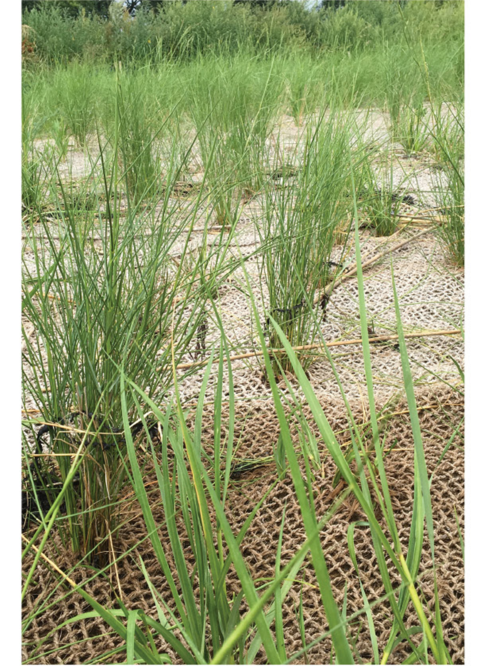
MARSH GRASS PLANTINGS INSTALLED WITH COIR BLANKET
