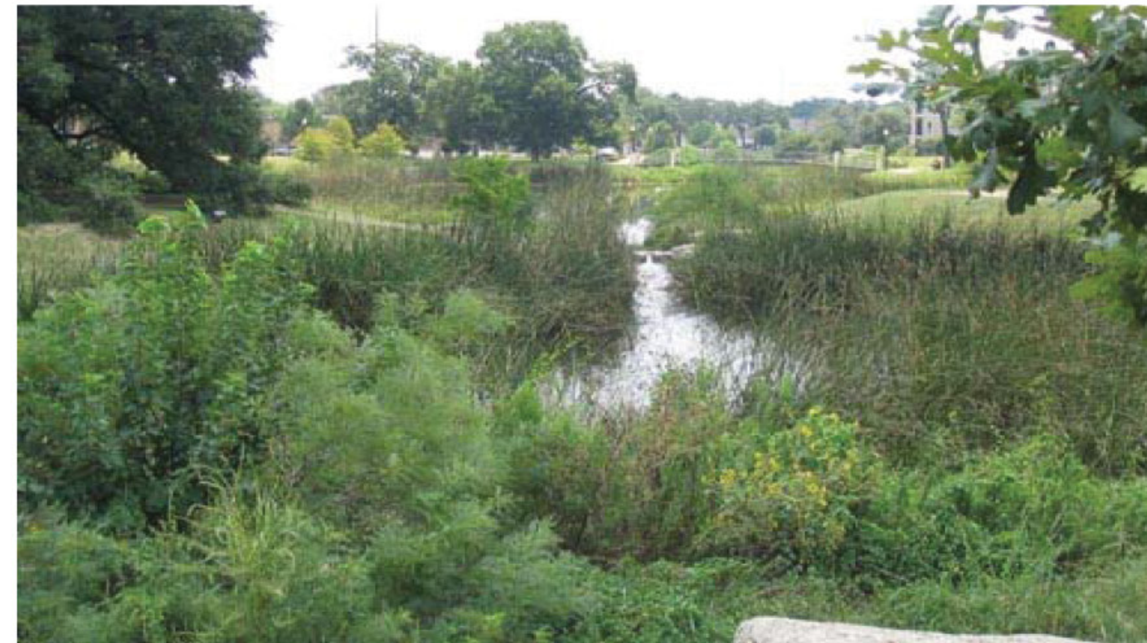
Bioretention basins increase stormwater filtering and infiltration
