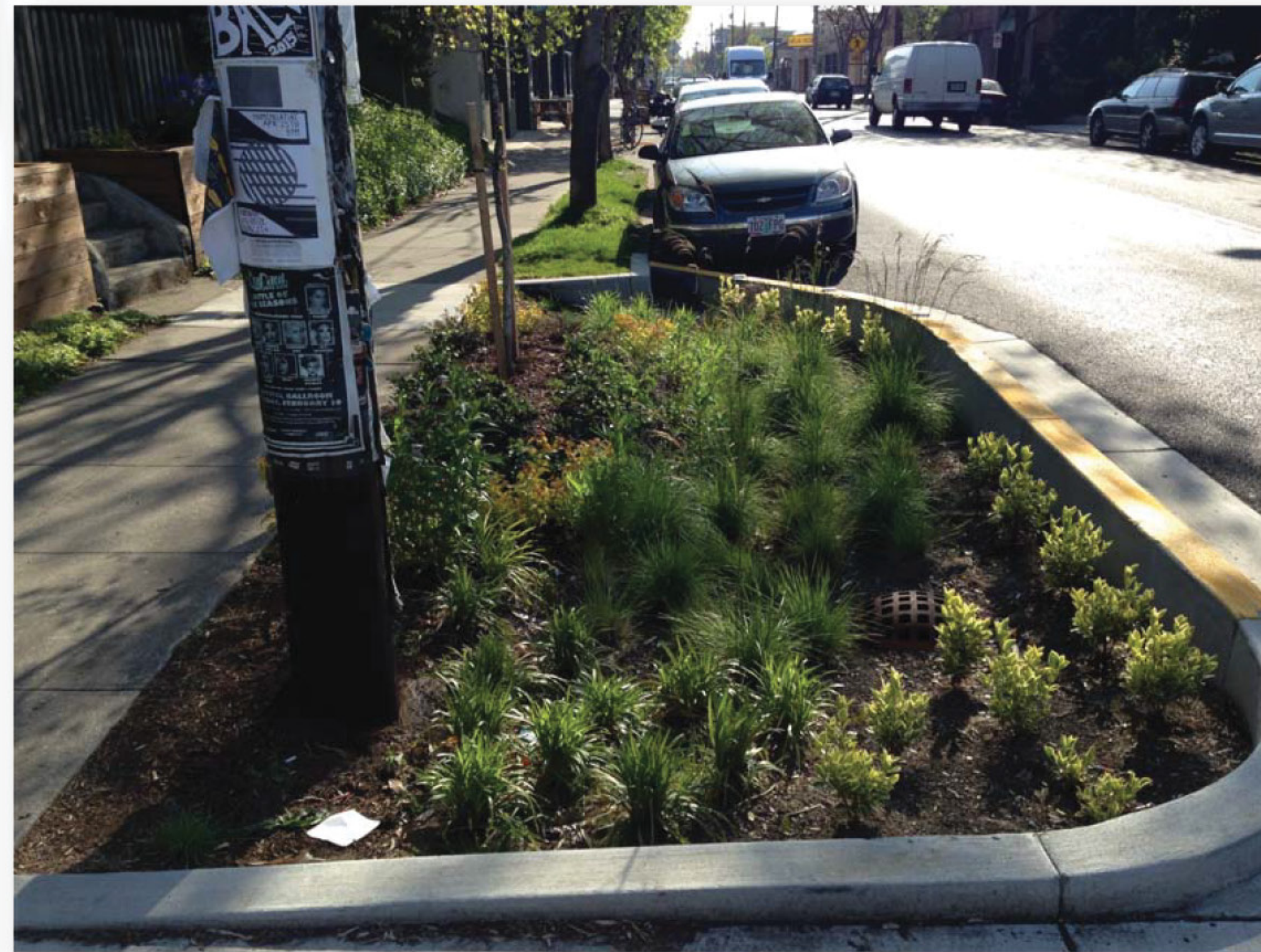
A Green Streets Recessed Stormwater Planter recently planted
