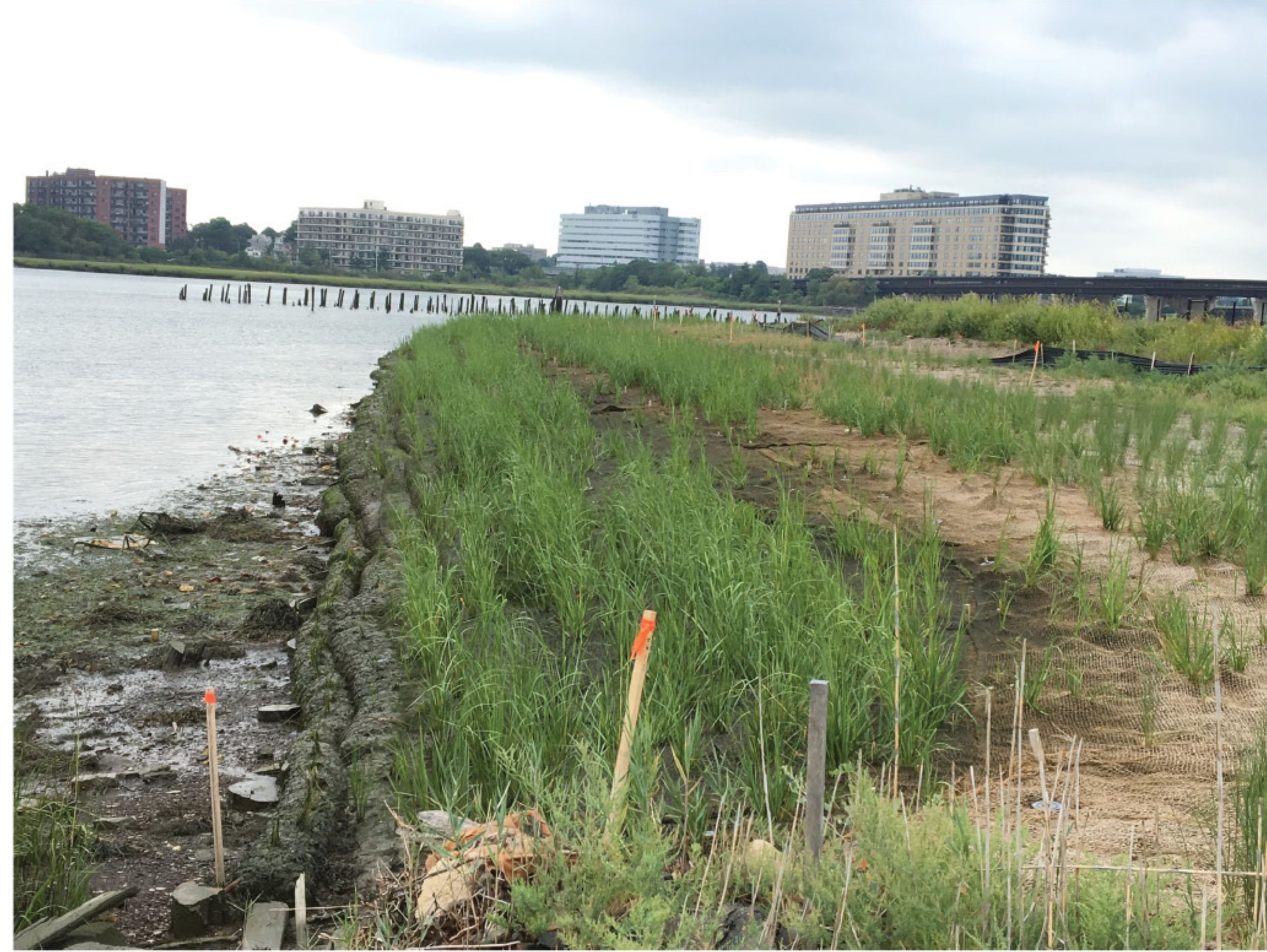
COIR LOGS & STRUCTURAL GEOTEXTILES
