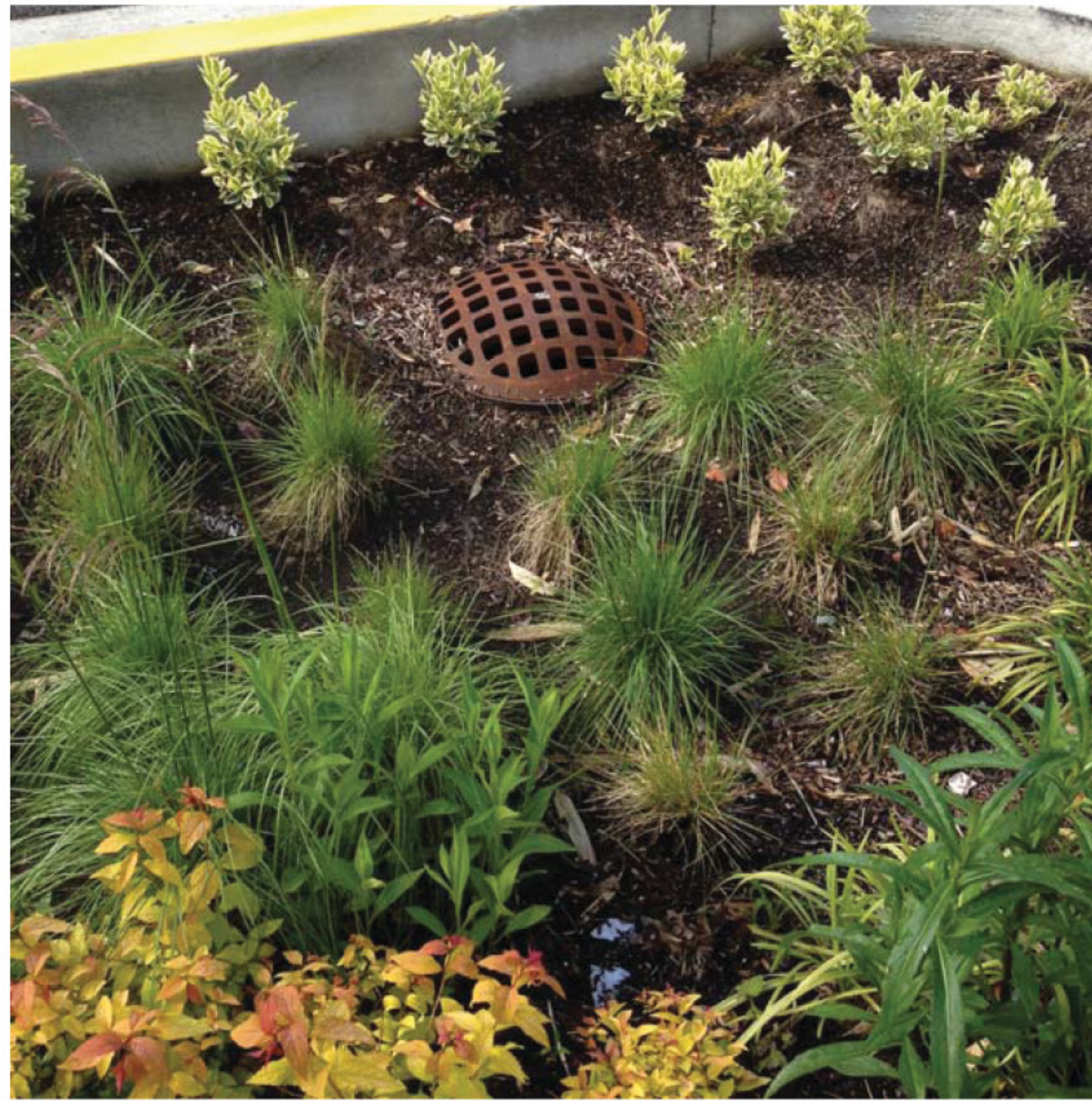
Bioretention basins increase stormwater filtering and infiltration
