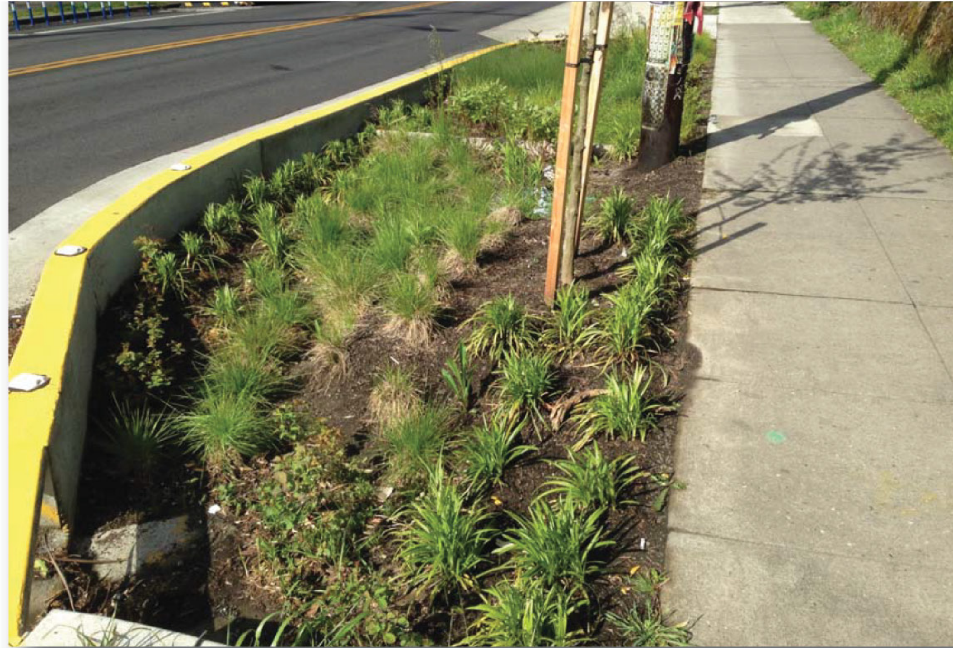
Recessed Stormwater Planters along Division Street | Portland Oregon
