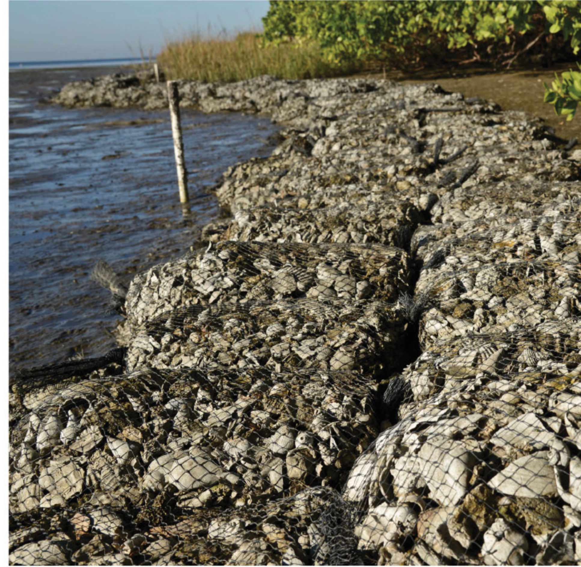
GABIONS WITH OYSTER SHELL AND ROCK
