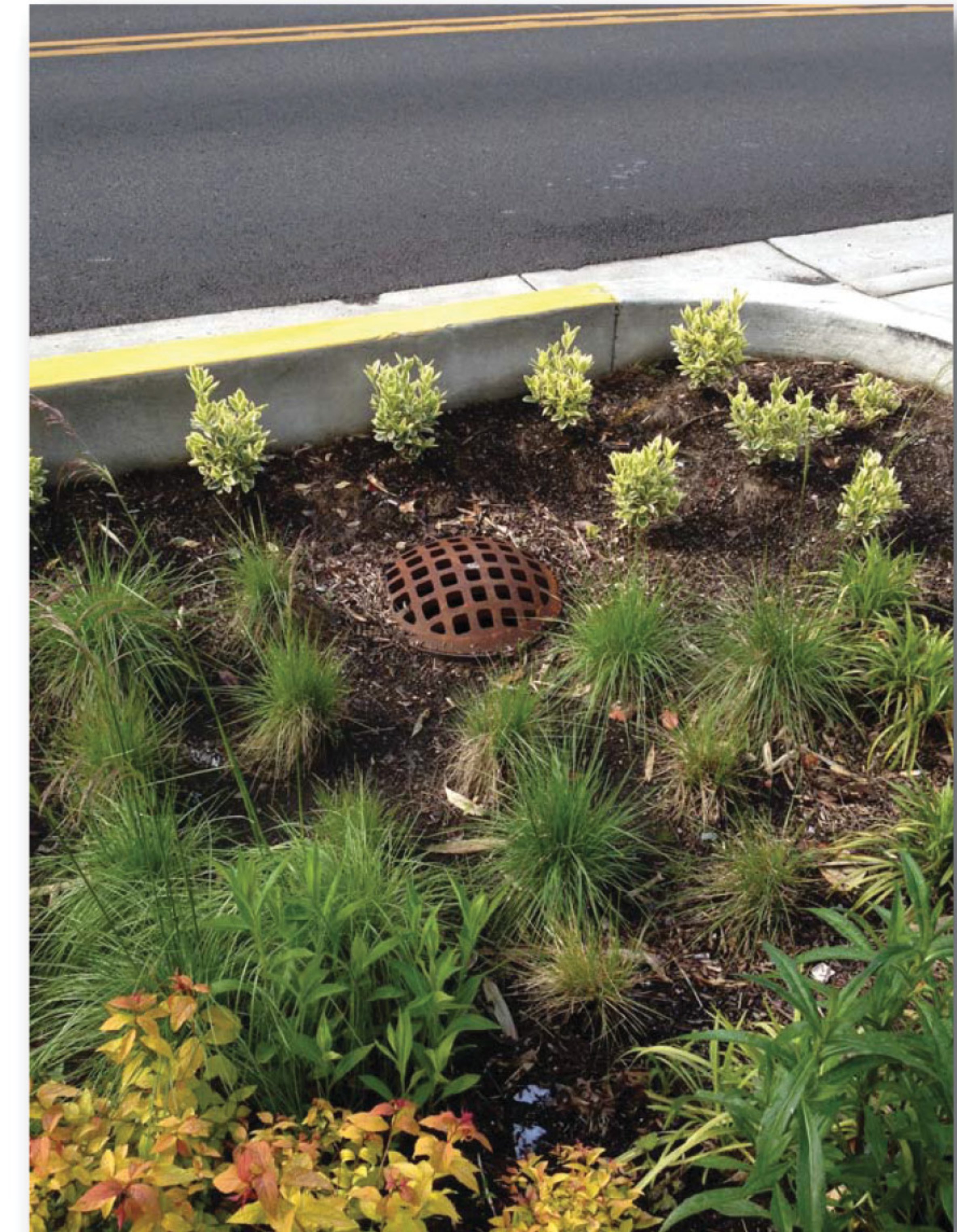
A bee-hive inlet is set at a high water level elevation and serves to decant stormwater to the street drainage system during extreme storms.
