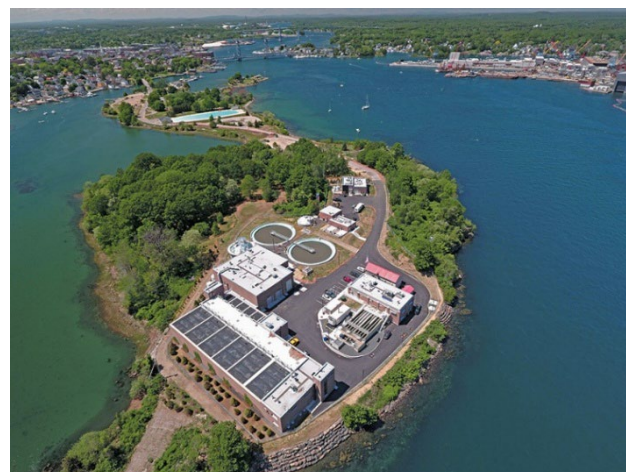
Figure 7. Aerial view of the Peirce Island Wastewater Treatment Plant
